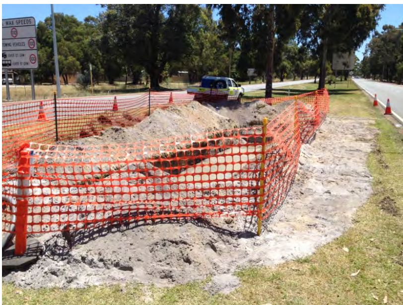
Figure H3: Infiltration Pit at Airport West Station
