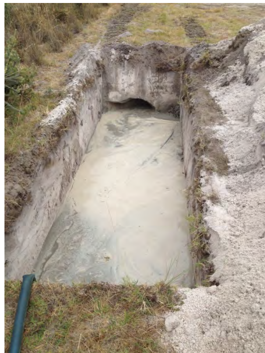
Figure H5: Infiltration Pit at Consolidated Station (left before discharge, right after start of discharge)
