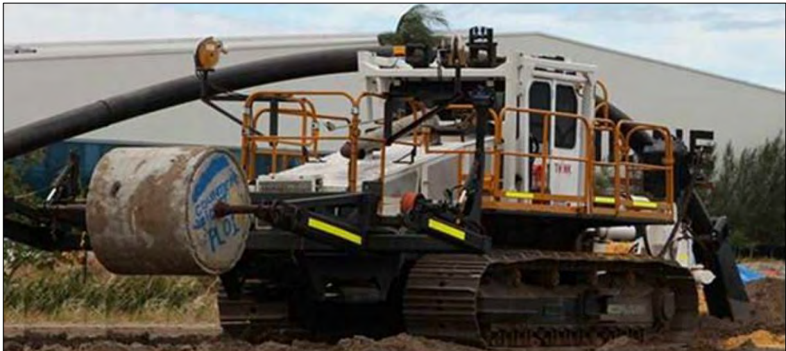
Figure 2: EcoPlough installing a PE pipeline
