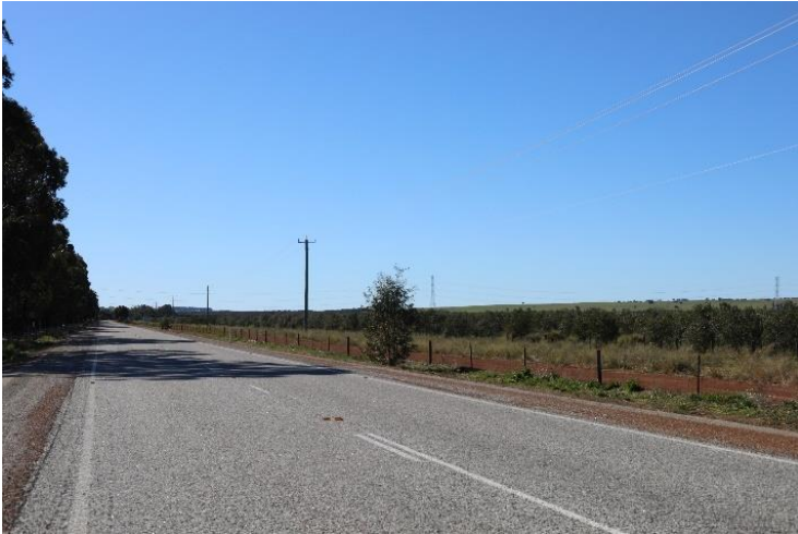
Figure 8-2 Transmissions lines in the middle ground, traversing orchard areas, Orange Springs Road, Orange Springs. (image: Aurecon, August 2025)
