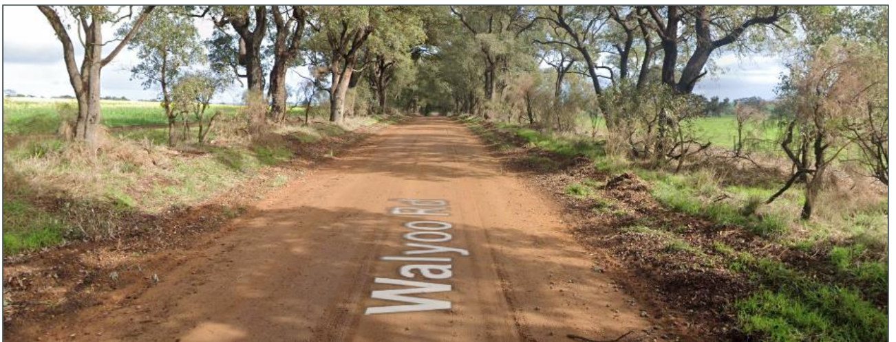
Figure 2-12 Walyoo Road looking west – Source: Google Street View, July 2023
