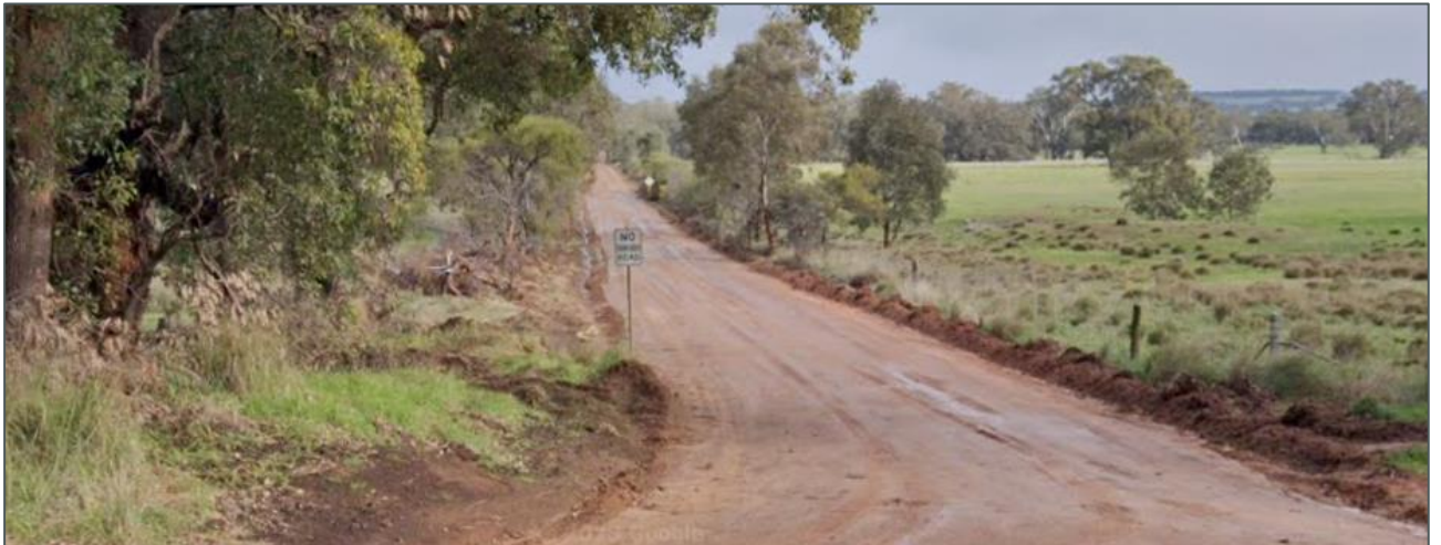
Figure 2-9 Walyer Walyer Road looking west – Source: Google Street View, July 2023
