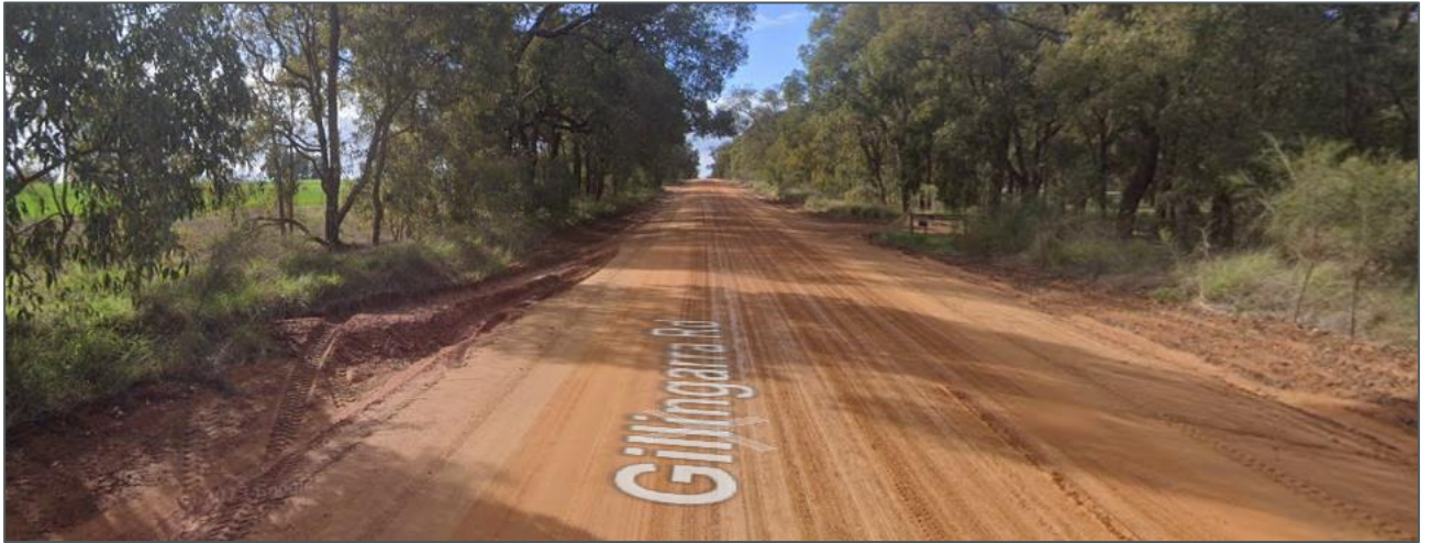
Figure 2-7 Gillingarra Road looking east – Source: Google Street View, July 2023
