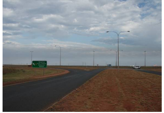
Photograph 4: Looking north-west on Great Northern Highway towards Port Hedland Road (GNH continues left)
