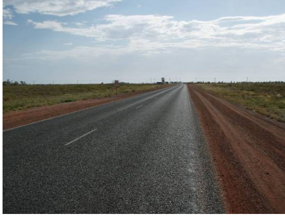
Photograph 3: Looking north-east on Great Northern Highway between Dalton Road and Pinga Street
