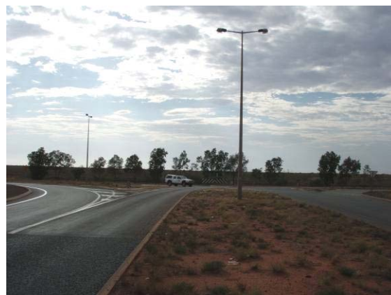
Photograph 2: Looking east on Great Northern Highway towards Wallwork Road (GNH continues left)
