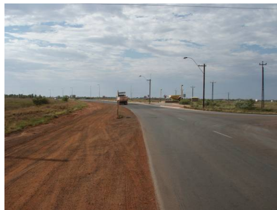
Photograph 8: Looking south on Pinga St between Cajarina Rd (on right) and Great Northern Hwy
