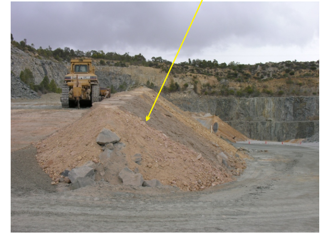
Construction of benches to enable backfill of the south eastern face
