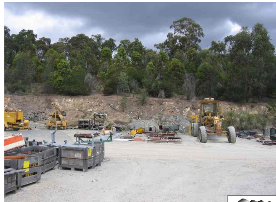
Figure 11 Lateral view of Area 1 rehabilitation. Compare to Figure 12
