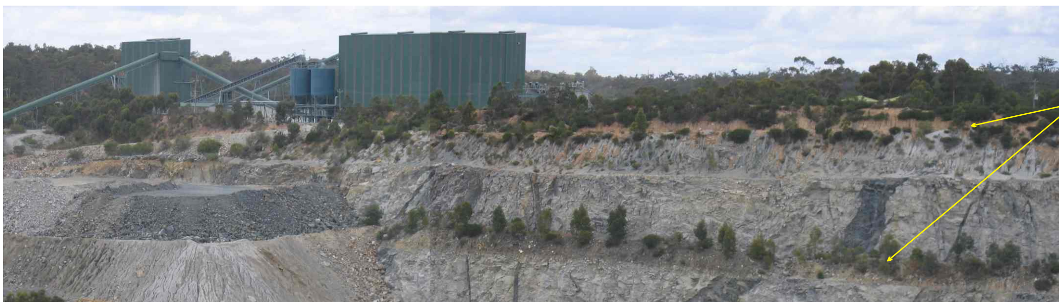
Figure 8 Southern face of the pit showing rehabilitation of the upper benches
