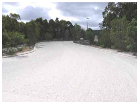
Figure 9A Entrance from Toodyay Road
