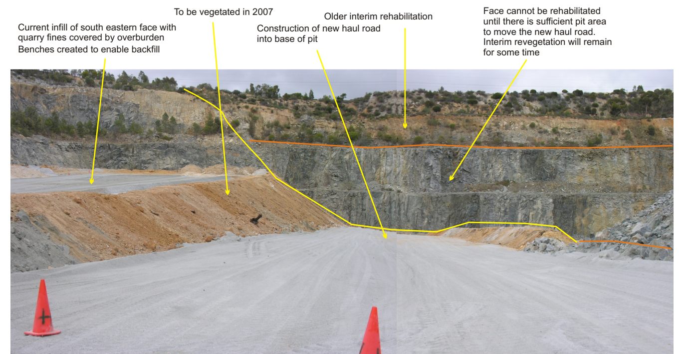
View south across the new area of backfill
