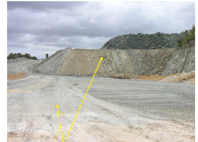
Construction of benches to enable backfill of the south eastern face To be covered by overburden and vegetate, to screen the diorite stockpile.
