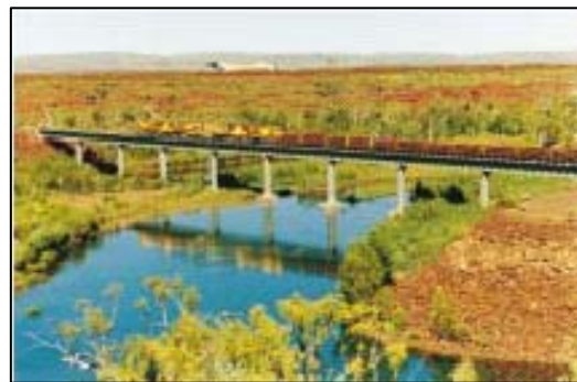
Existing rail infrastructure
