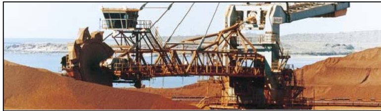
Stacker-reclaimer at Cape Lambert
