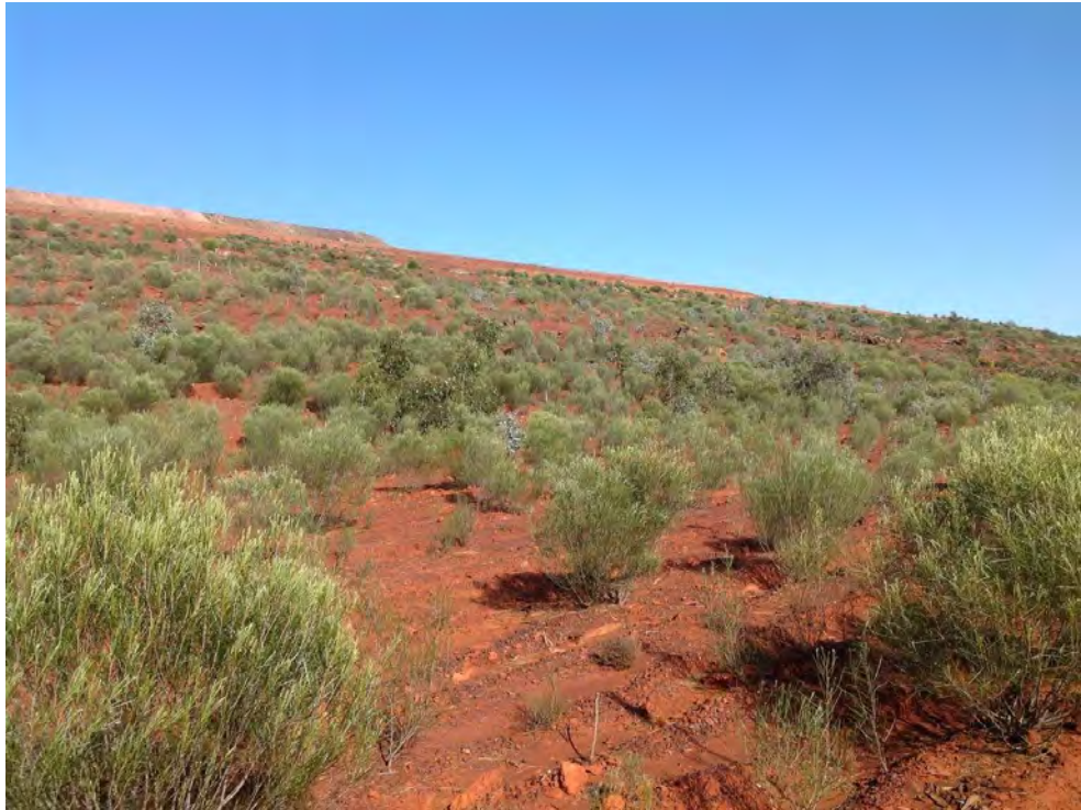
Figure 3-29 Rehabilitation at the approved Koolyanobbing Range Mine Operations. The image depicts the progress of rehabilitation (at approximately 3.5 years age) at the Koolyanobbing Range B/C Deposits Waste Rock Landform. Progressive rehabilitation works has been completed on the lower lifts of the B/C Deposit Waste Rock Landform, with the active construction of the upper lifts also visible. Source: Globe Environments, September 2015.
