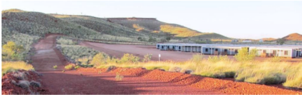
The width between firebreaks surrounding the Japal Camp does not meet Local Government requirements and is too narrow to effectively reduce bushfire risk.
