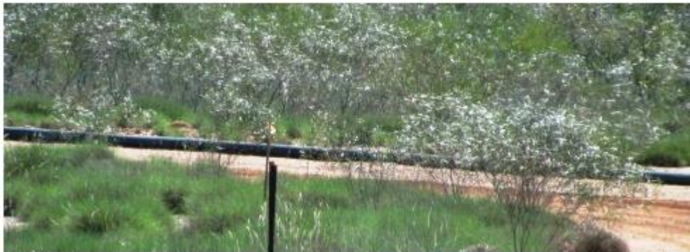
Plastic pipes leading to the concentrate handling facility are exposed to damage from vegetation that will burn intensely during bushfire.
