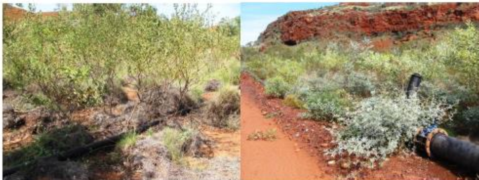
Potable water (left) and critical raw water pipes (right) are exposed to damage from vegetation that will burn intensely during bushfire.
