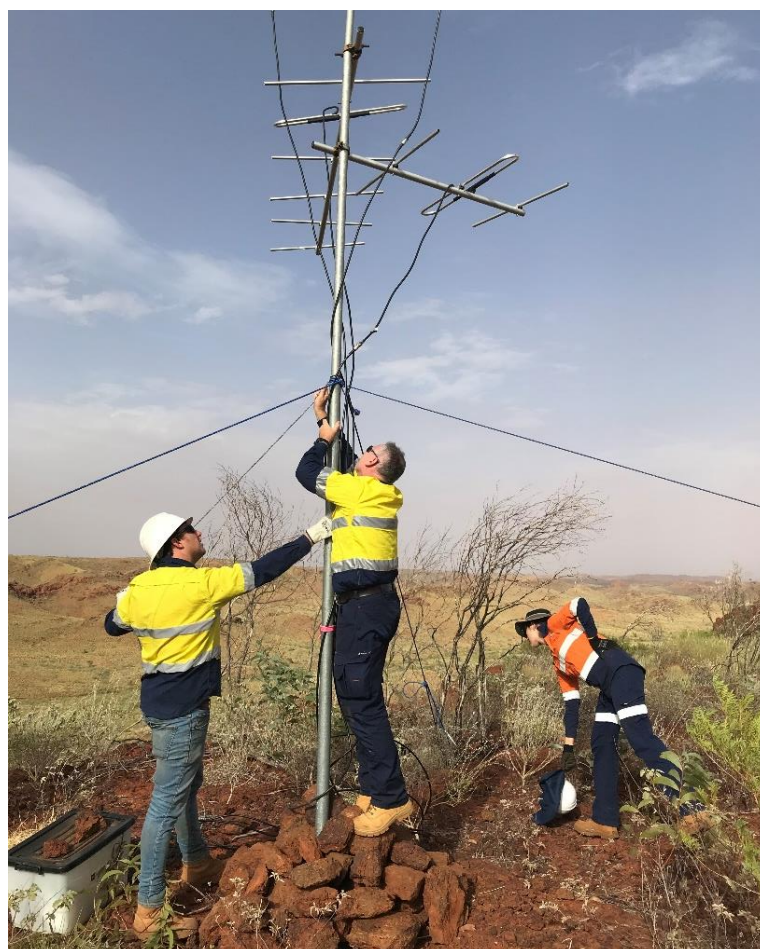
Plate 9: Maintenance of base station 5 north-west
