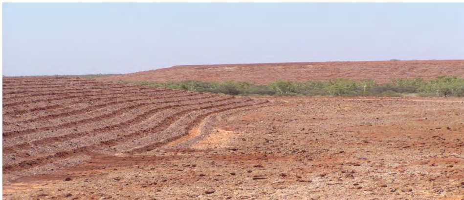
Figure 13: Contour ripping on freshly completed reprofiling
