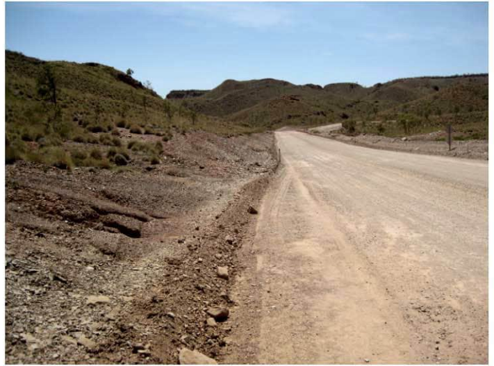
16. Cut shale / siltstone on South road side
