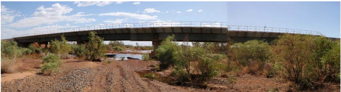
Photo 2 - BHP Rail Crossing At Chinnamon Creek
