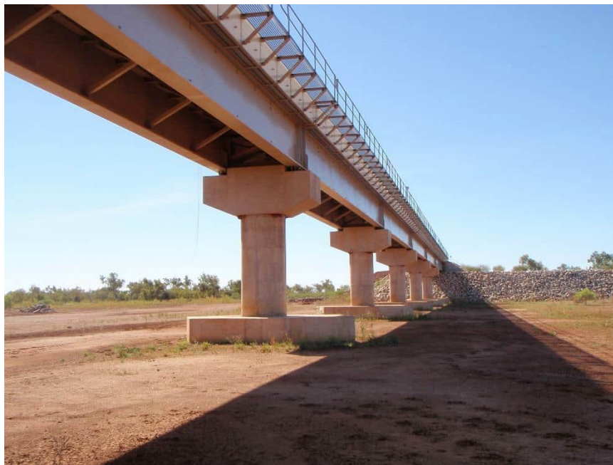
PHOTO 3 - ROY HILL RAIL CROSSING
