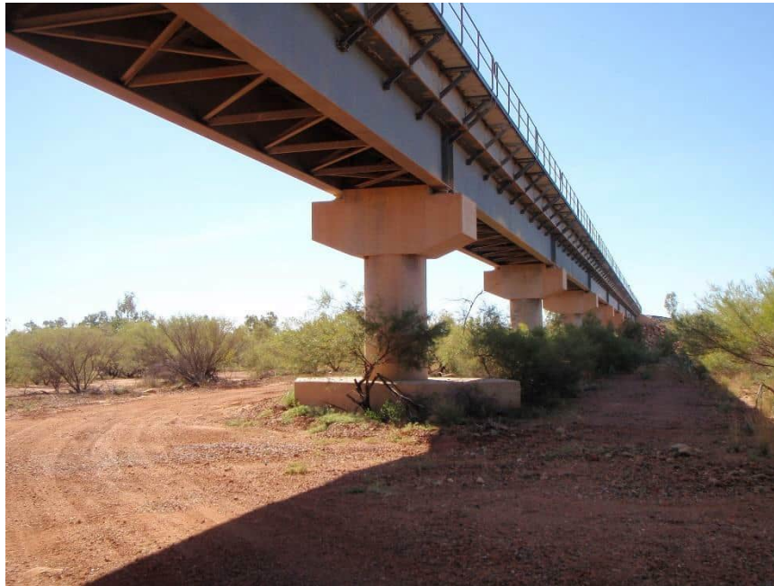
PHOTO 2 - FMG RAIL CROSSING
