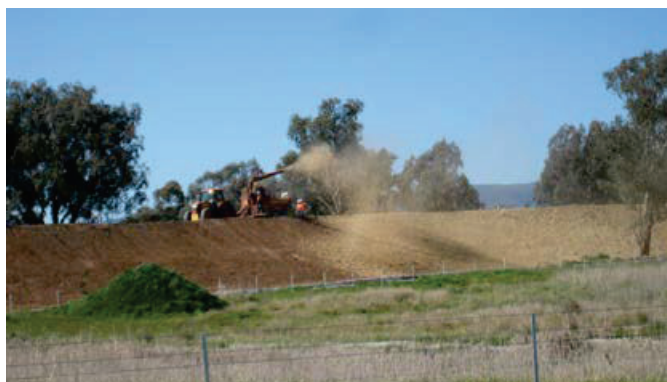
Figure FS6a: Straw mulch being applied with a trailer mounted straw blower.
