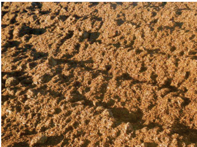
Figure FS8a: Correctly applied BFM Hydromulch – note 100% coverage. (Source: Landloch Pty Ltd)
