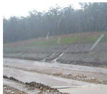
Figure 3.2c: Concentrated flow on a batter during a heavy rain event.
