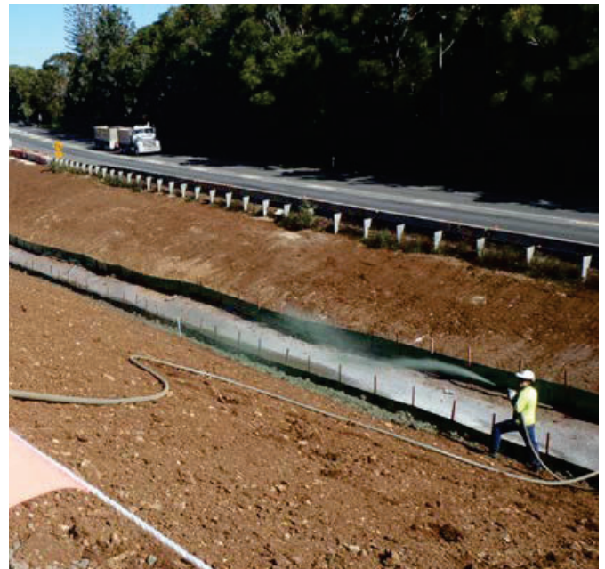
Figure FS5a: Hydroseed application on a prepared batter.
