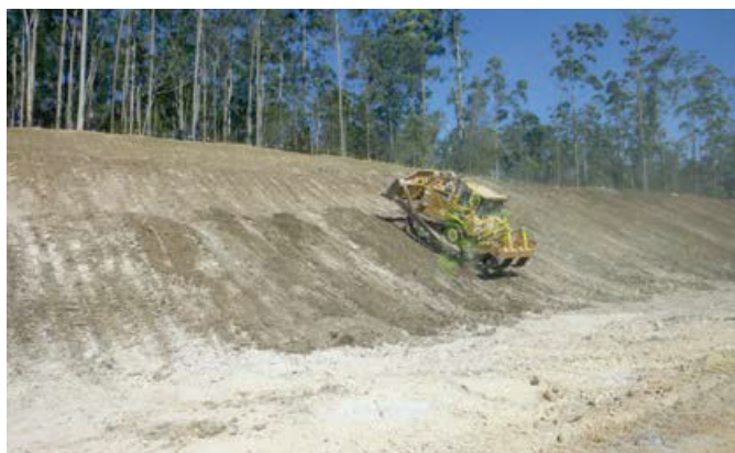
Figure 3.13b: Track rolling a batter in preparation for the application of a stabilisation technique.
