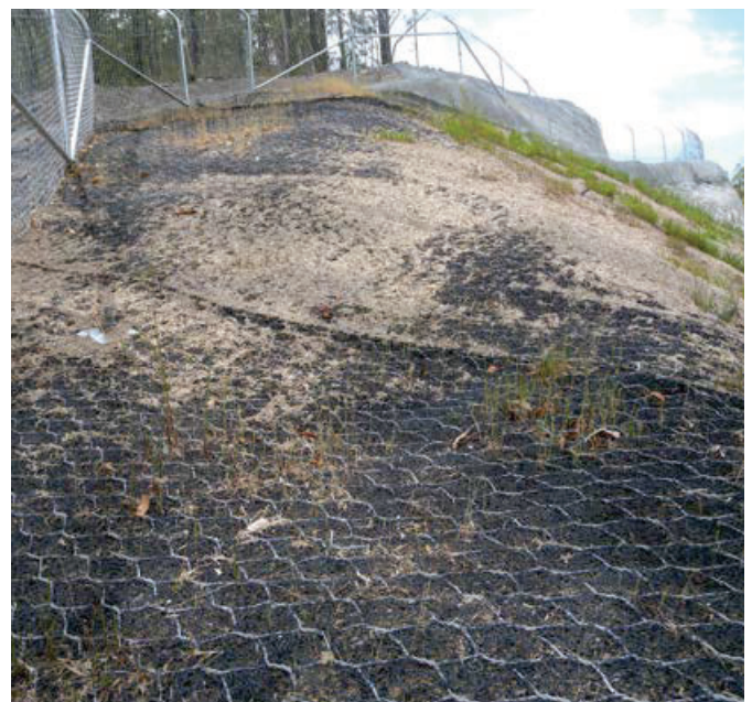
Figure FS15b: Non-soil filled turf reinforcement mat.
