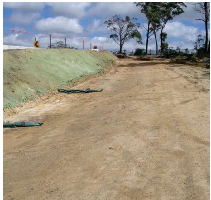
Figure FS3a: Tackifier applied with a green dye.
