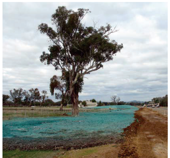
Figure FS7b: Hydromulch application on a shallow gradient batter, with green dye for visibility.
