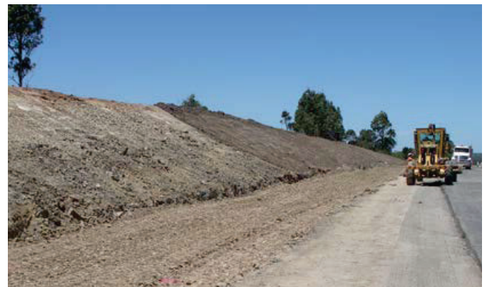
Figure 3.1.1: Topsoil being progressively applied over a prepared batter.
