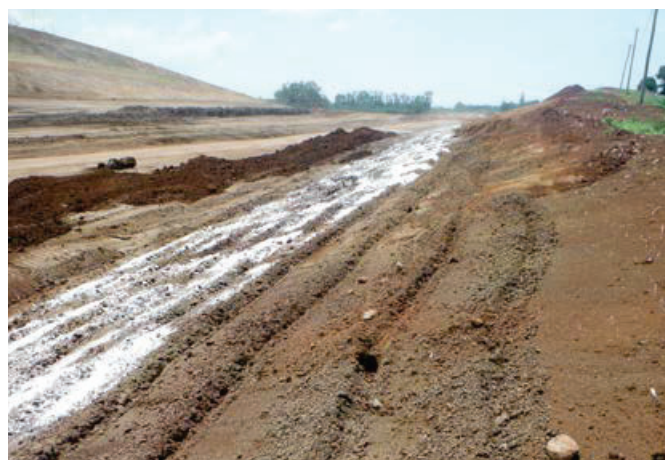
Figure 3.13d: Contour scarification across a batter. Lime amelioration is being applied prior to topsoil application.
