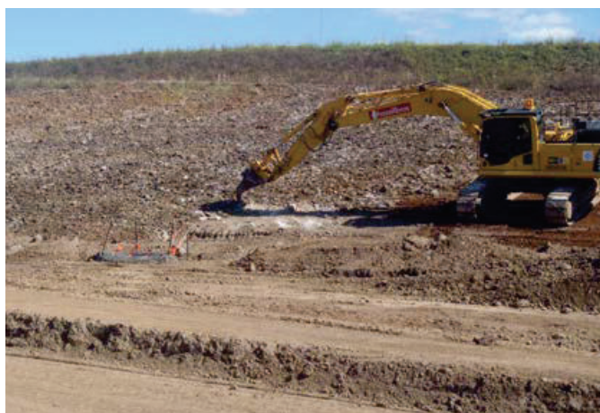
Figure 3.13a: Contour ripping across a batter using an excavator. Note that on batters \leq 3h:1v this can also be done with a bulldozer.
