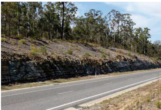
Figure FS4a: Mix of 60% soil and 40% shredded mulch from local vegetation at Glenugie Upgrade on rock cutting.
