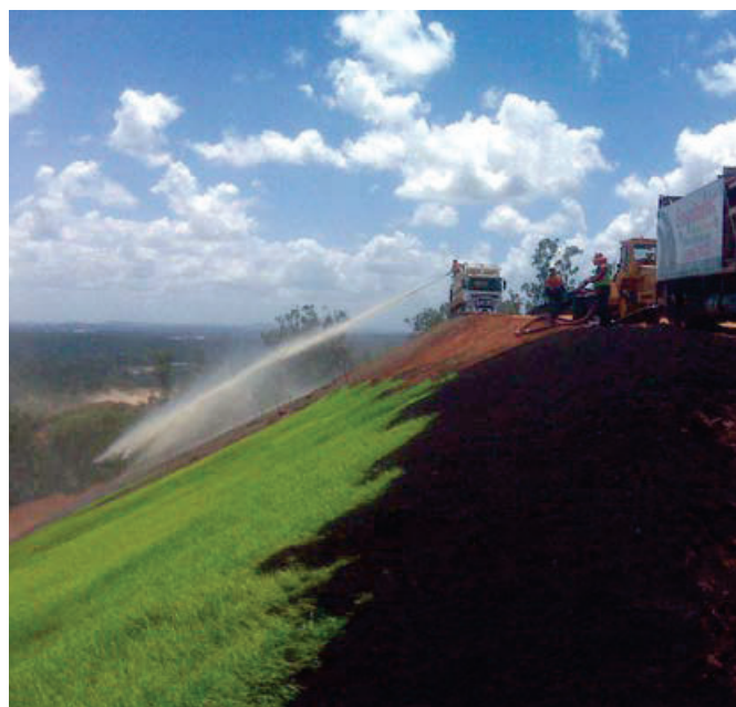
Figure FS13 b: Watering of compost blanket after application. (Source: The Hills Bark Blower)
