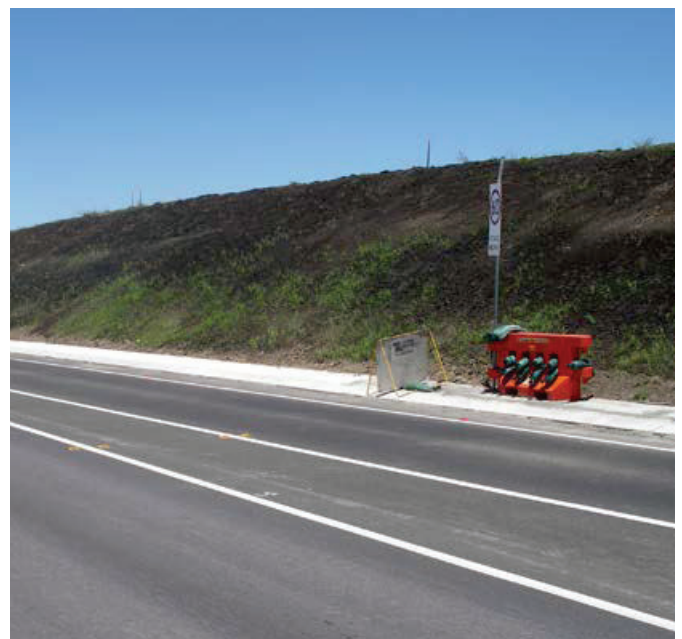
Figure FS2b: Uneven establishment of grass through bitumen emulsion.
