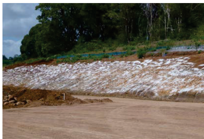
Figure 3.5.2b: Lime applied to a batter waiting to be incorporated.
