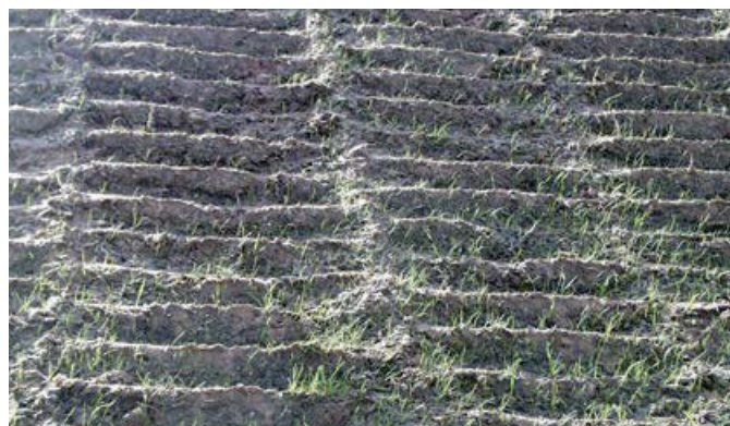
Figure 3.5.2a: Track rolled batter with horizontal scarification, and seed beginning to germinate.
