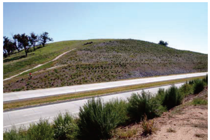
Figure FS4b: Woodchip and shredded mulch from local paper mill on planted 2h:1v cuts at Woomargama Bypass.
