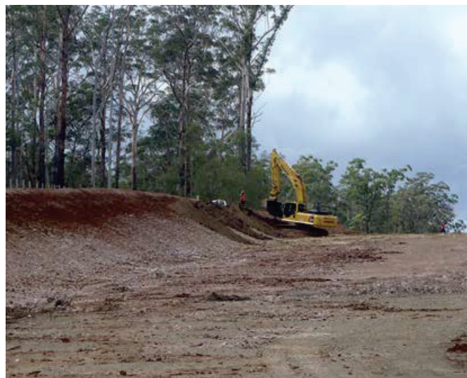
Figure 3.3a: Topsoil being re-applied to a batter, after it was stripped and saved during the construction process.
