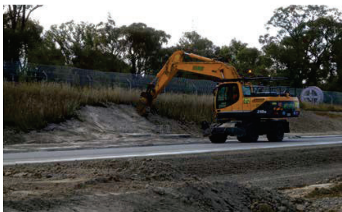
Figure 3.13c: Pad roller preparing a batter in preparation for the application of a stabilisation technique.
