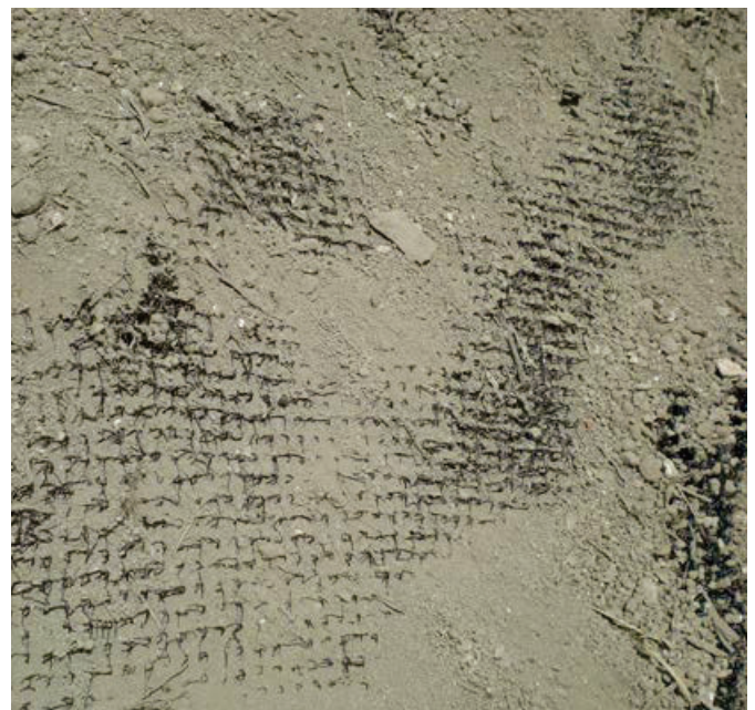
Figure FS15a: Soil-filled turf reinforcement mat. (Source: Wally Butman – Profile Products)
