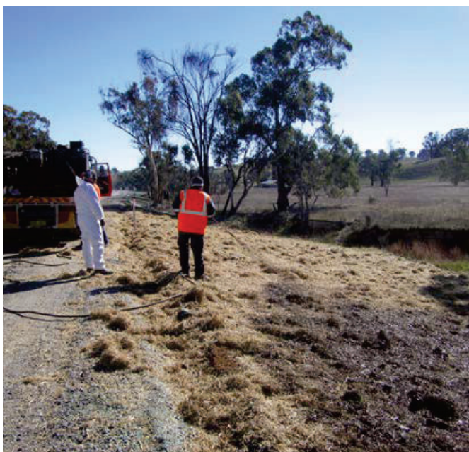
Figure FS2a: Application of bitumen emulsion (darker area) over straw mulch.
