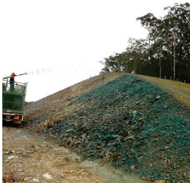
Figure FS9a: Application of Hydrocompost on the Kempsey Bypass. (Source: Matthew Easton)
