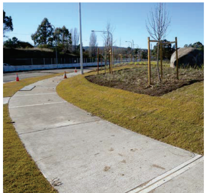
Figure FS14b: Turf placed on variable slopes, Bega Bypass.
