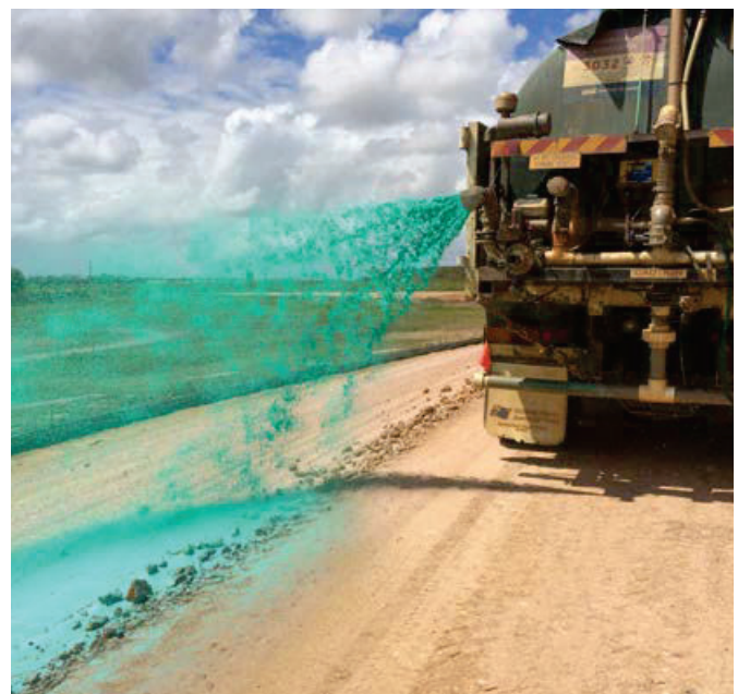
Figure FS3b: Water cart application of a tackifier. (Photo: Vital Chemical Pty Ltd)
