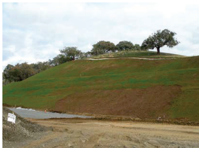
Figure 3.1.2a: A large batter slump due to insufficient batter preparation.
