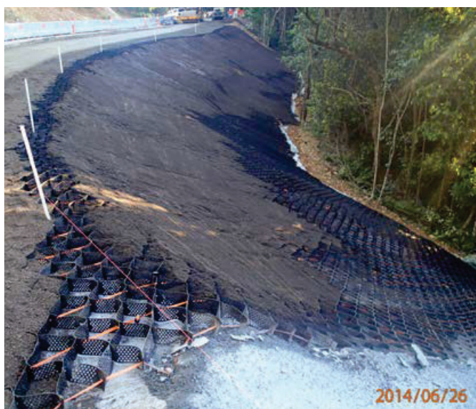
Figure FS12a: Installation of cellular confinement system – backfilling with unbound granular material beneath the pavement and imported topsoil on the batter slope. (Source: Queensland Department of Transport and Main Roads)
