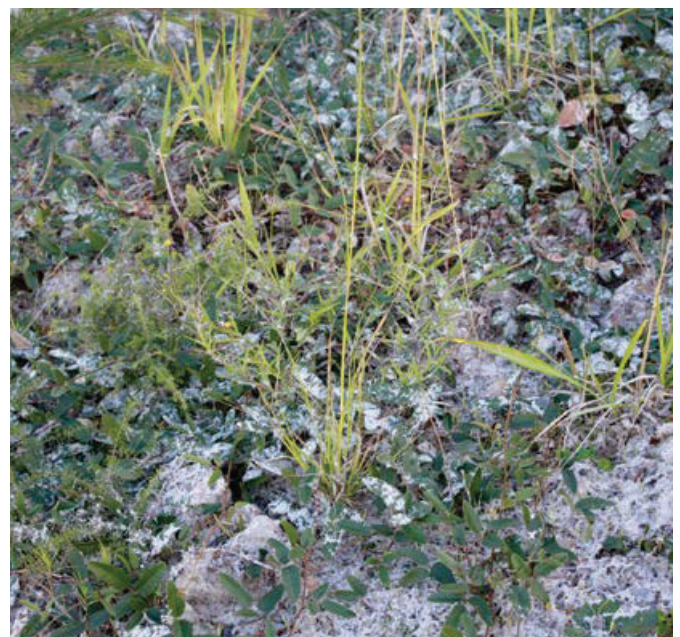
Figure FS5b: Diverse vegetation establishment resulting from hydroseeding overlaid with hydromulch on the Kempsey Bypass.
