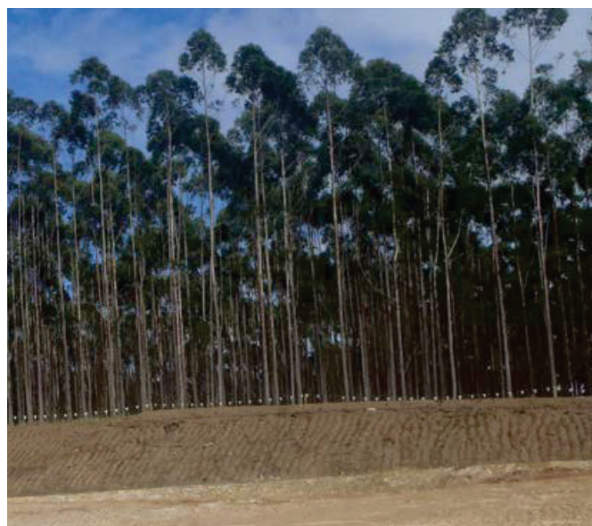
Figure 3.1.2b: A batter that had been incorrectly vertically scarified during construction, creating preferential flowpaths for runoff, which has started causing rill erosion.
