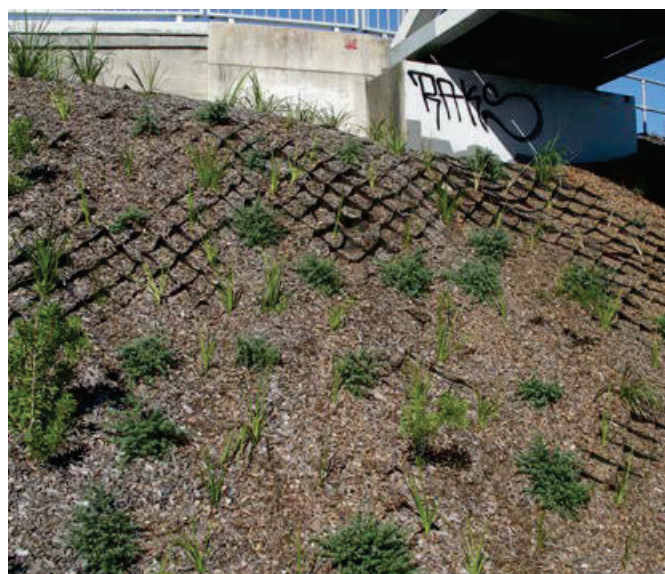
Figure FS12b: Cellular confinement that has been installed and planted out on an extremely steep slope, and begun to slump due to insufficient anchoring.
