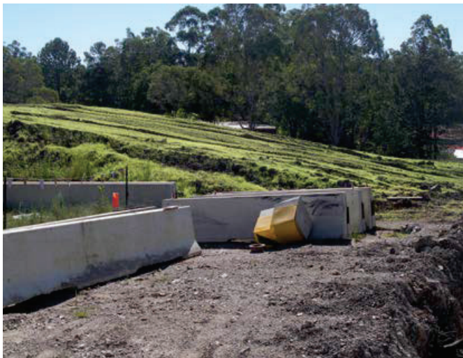
Figure 3.5.4: Topsoil stockpile that has been set up to allow machinery to apply and incorporate ameliorants.
