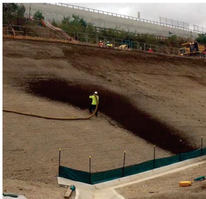
Figure FS13a: Application of a compost blanket on a steep batter. This application also included the addition of woodchip to provide additional erosion protection. (Source: Leighton Contractors)
