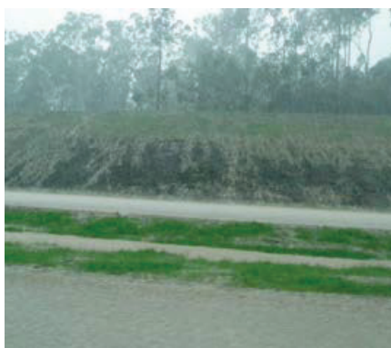
Figure 3.2b: Sheet flow over batter, Pacific Highway, Glenugie Upgrade.
