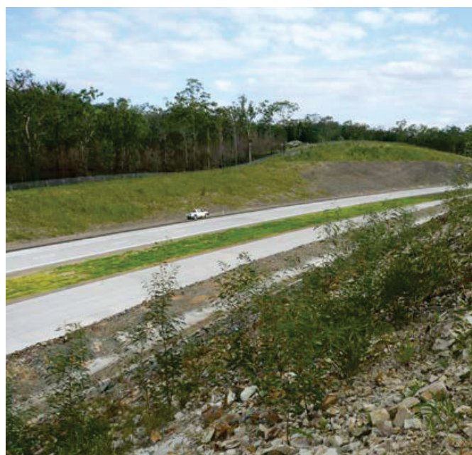
Figure FS9b: Vegetation establishment from Hydrocompost on the Kempsey Bypass. (Source: Matthew Easton)
