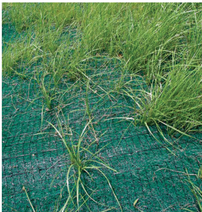
Figure 3.11: Effective soil surface cover, provided by a combination of Turf Reinforcement Mat and seeded grass that has begun to establish through it.
