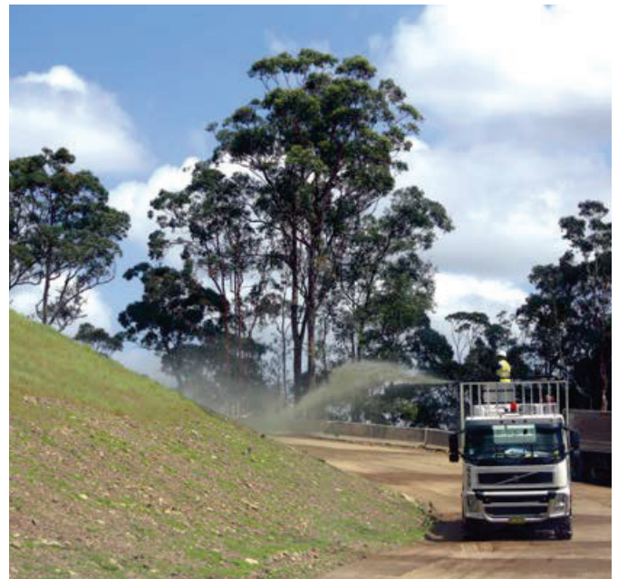
Figure FS7a: Standard Hydromulch being applied to a batter on the Hunter Expressway.
