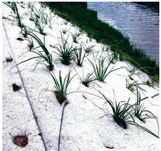
Figure FS11a: Erosion control blanket with cuttings for plantings. (Source: Geofabrics Australasia Pty Ltd)
