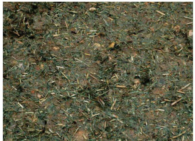
Figure FS8b: Poorly applied BFM Hydromulch – note ineffective coverage. (Source: Landloch Pty Ltd)
