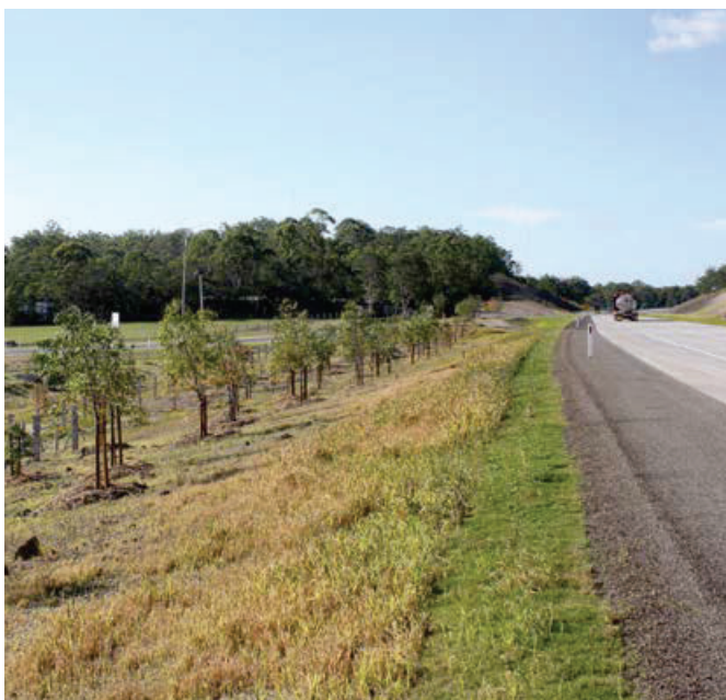
Figure FS14a: Turf strip at top of seeded batter to spread sheet flow, Kempsey Bypass.
