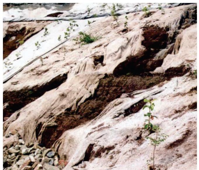
Figure FS10b: ECB failure due to poor surface preparation and water ingress through tree planting cuts. (Source: Landloch Pty Ltd)
