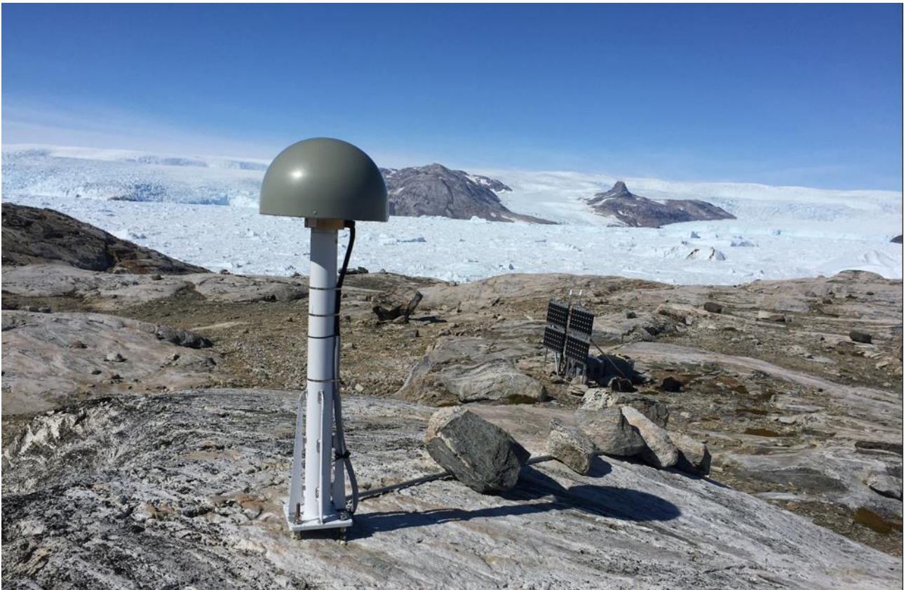
Figure 9-1 - Example CORS that would be representative of that required for the subsidence monitoring program. Equipment would be mounted to a single pole. (Source – Unavco)
