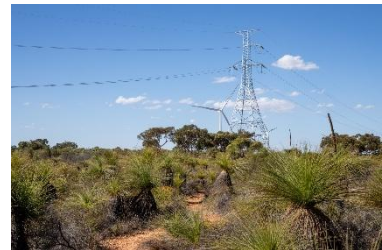
Yandin Wind Farm and OHTL viewed from the Yandin Lookout walking trail
