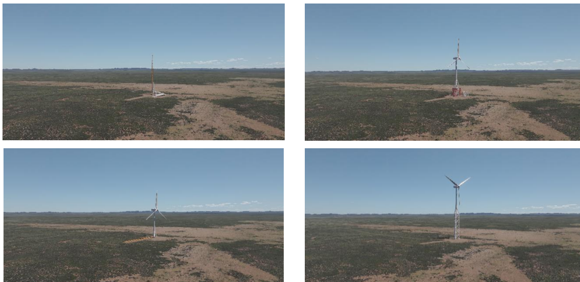
Plate 3-1: Nabralift Tower Construction
