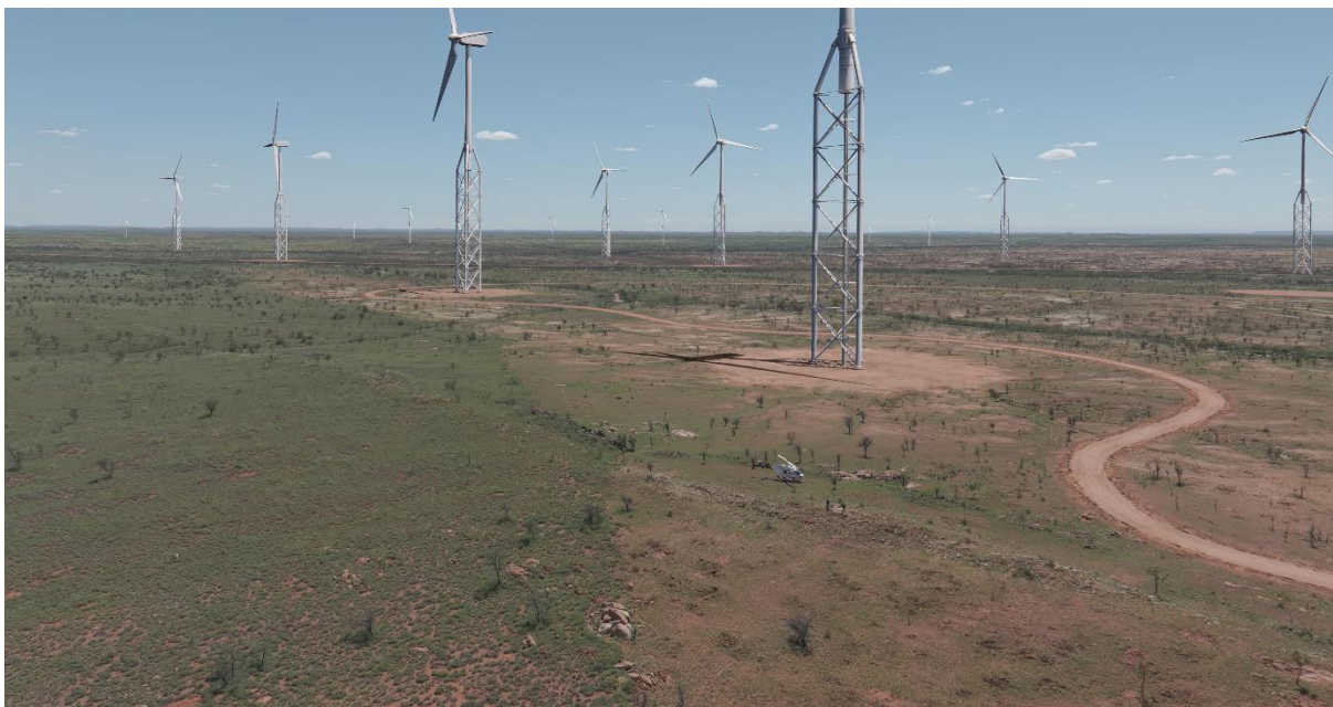
Plate 3-3: Access roads to the Generation Hub area
