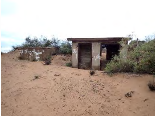
Plate 4. Historical structures within Project Area
