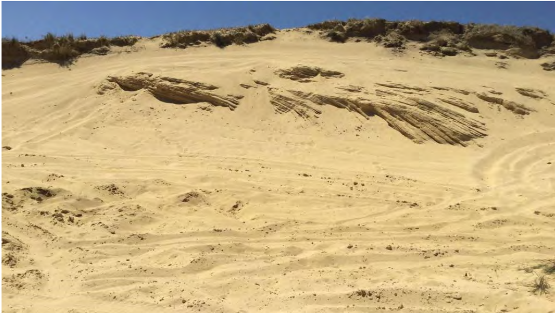
Figure 5-3: LS4 (Cemented Safety Bay Sand) exposed as subcrop in cutting, exhibiting planar cross-bedding typical of aeolianites
