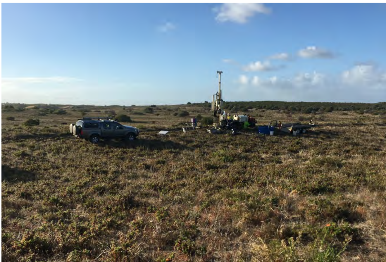
Alkimos Station Drill Site
