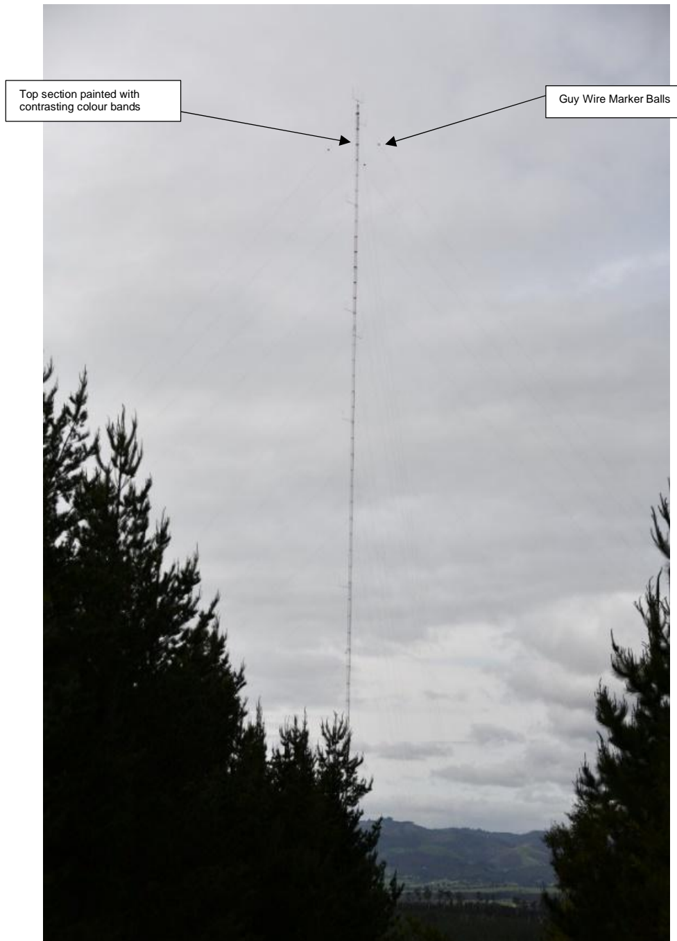
Figure 8 – An appropriately marked Meteorological Monitoring Mast 22
