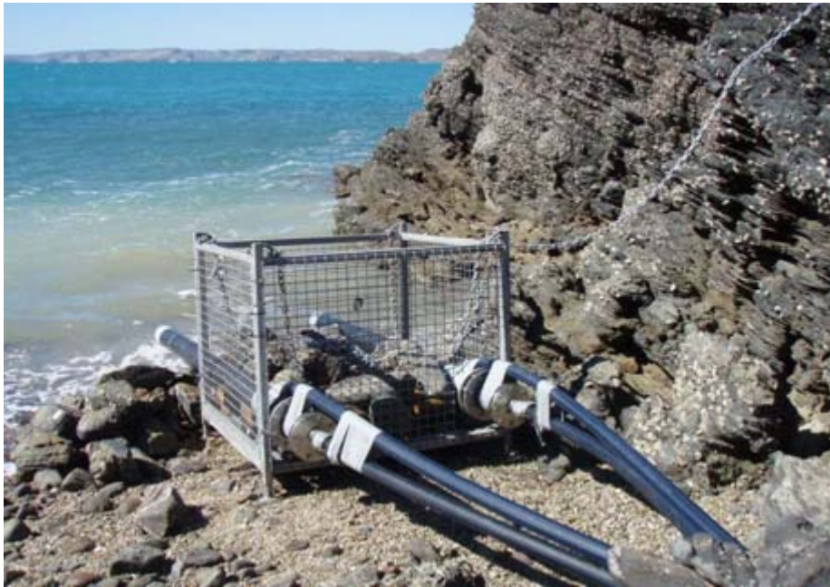
Plate 8 Desalination saltwater inlet during installation
