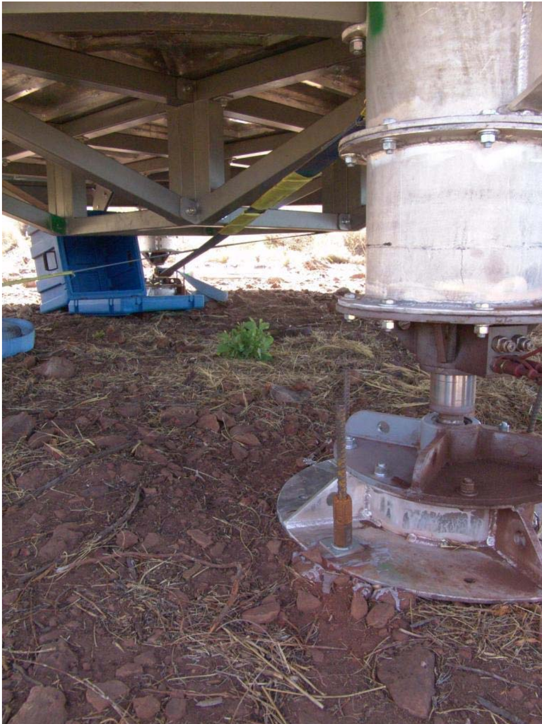
Plate 13 Ground disturbance underneath the Universal Drilling Platforms shown restricted to anchoring feet (vegetation regrowth at ~6 weeks)
