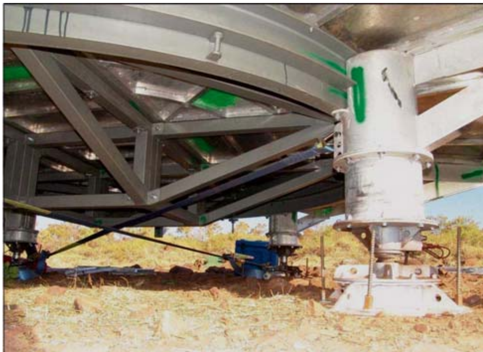
Plate 11 Close-up of Universal Drilling Platform support leg and anchor points
