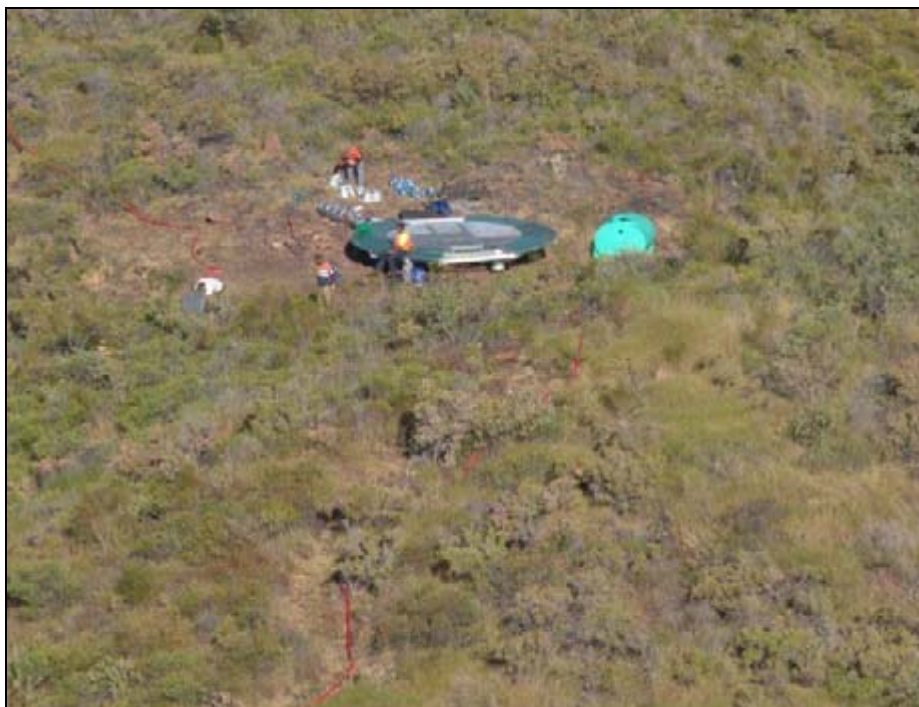
Plate 9 Universal Drilling Platform, walking track, water circulation pipe and main reservoir tank
