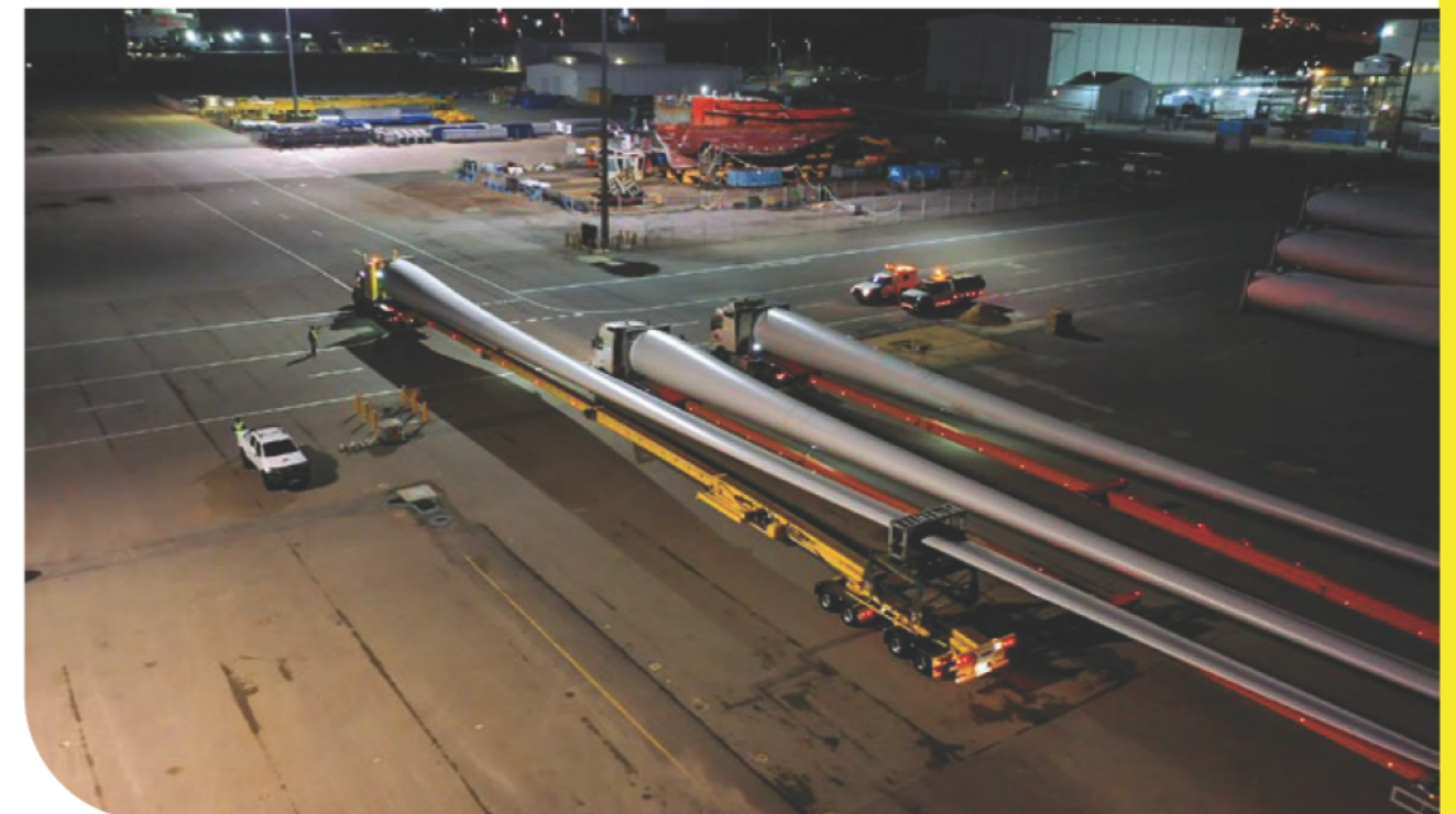
Above: Extendable blade trailers loaded with 75m blades for the Yandin project in Western Australia.
