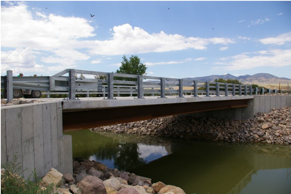
Plate 1: Example of a span bridge
