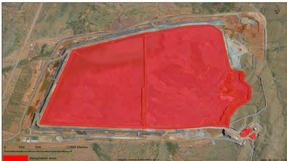
Figure 10-13: Designated area at Tailings Storage Facility
