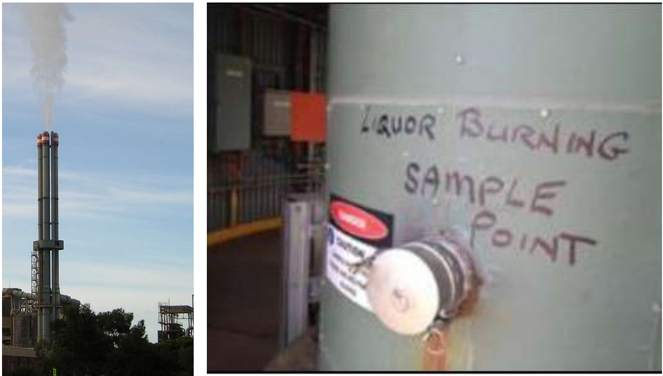
Figure 12: (a) Liquor burner stack (in multi-flue) and (b) Liquor burner sampling point
