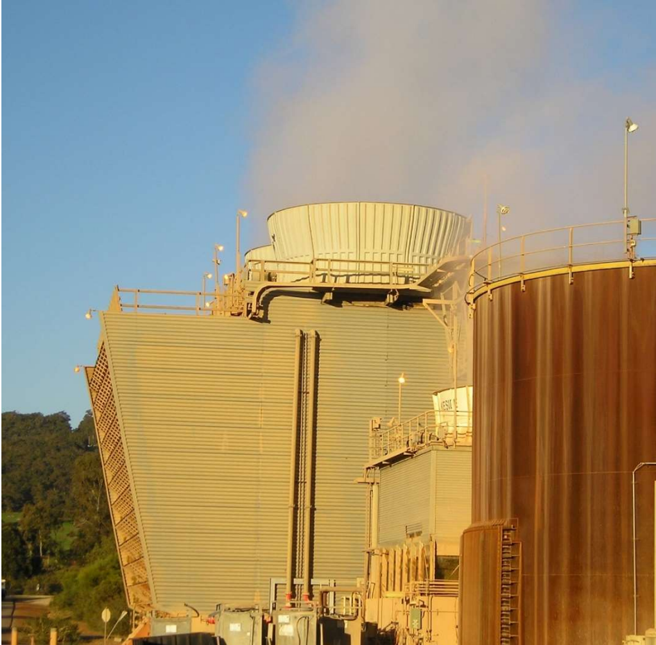
Figure 9: Precipitation Cooling Towers
