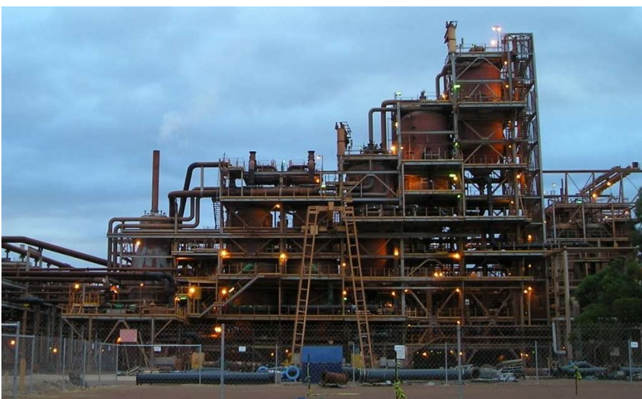
Figure 3: Digestion and 30-2 containment tank stack
