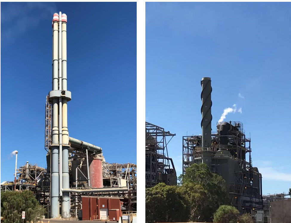
Figure 14: (a) Calciner 1-3 multi-flue stack and (b) Calciner 4 stack
