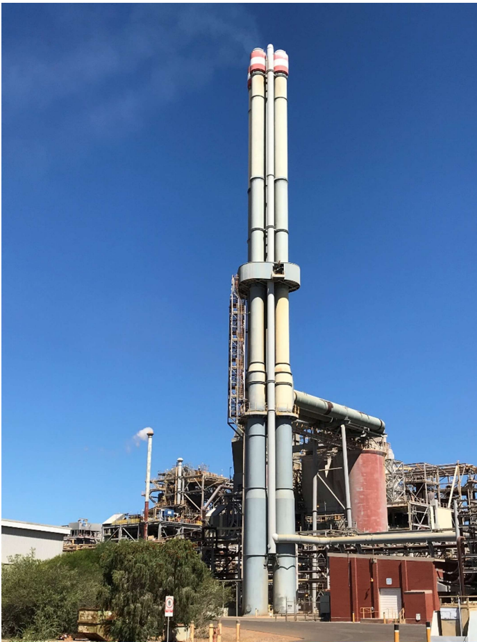
Figure 16: Calcination multi-flue stack (includes Calciner 1-3 LVV)
