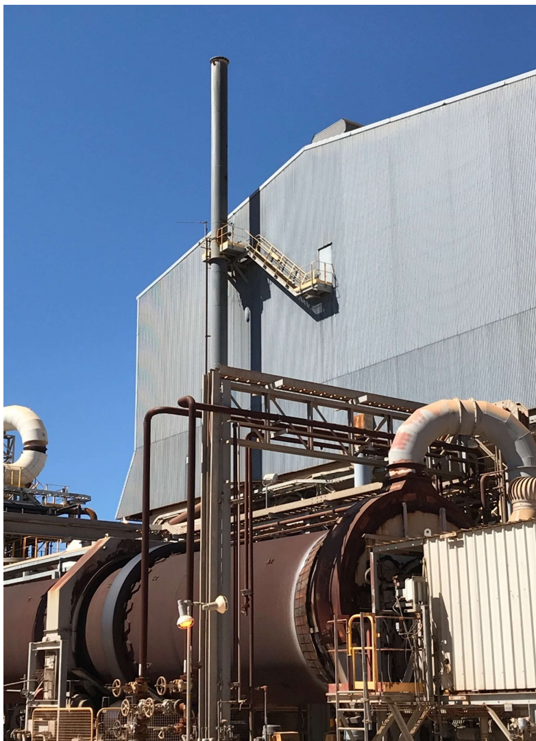
Figure 11: Oxalate filter press building stack (47K1)
