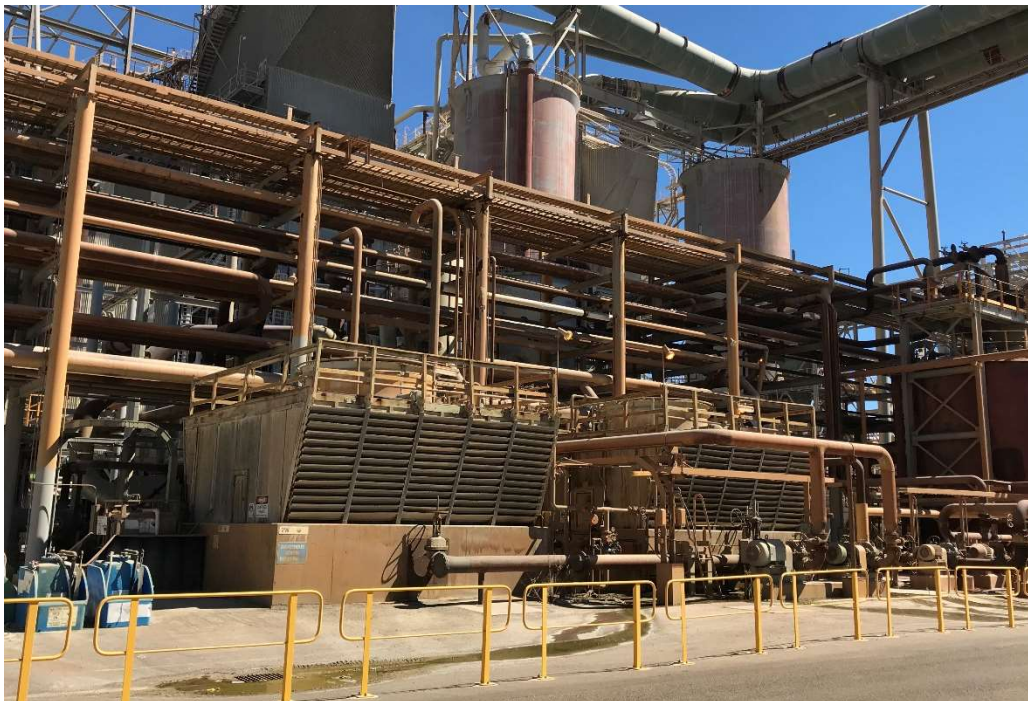
Figure 19: Calcination cooling towers
