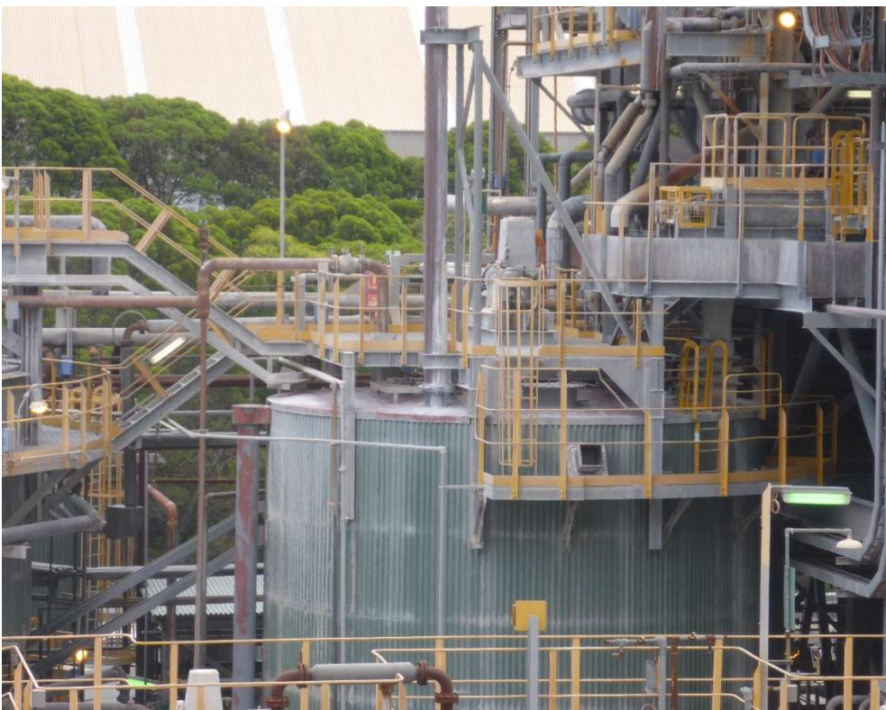
Figure 13: Liquor Burning Slurry Mixing Tank (48A)
