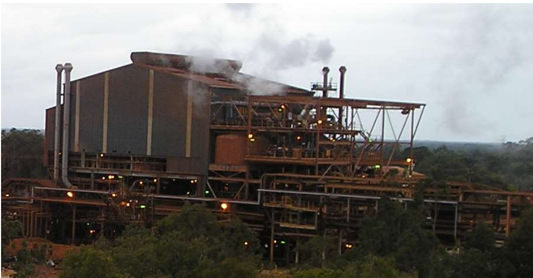
Figure 4: Sand Separation (Building 26)
