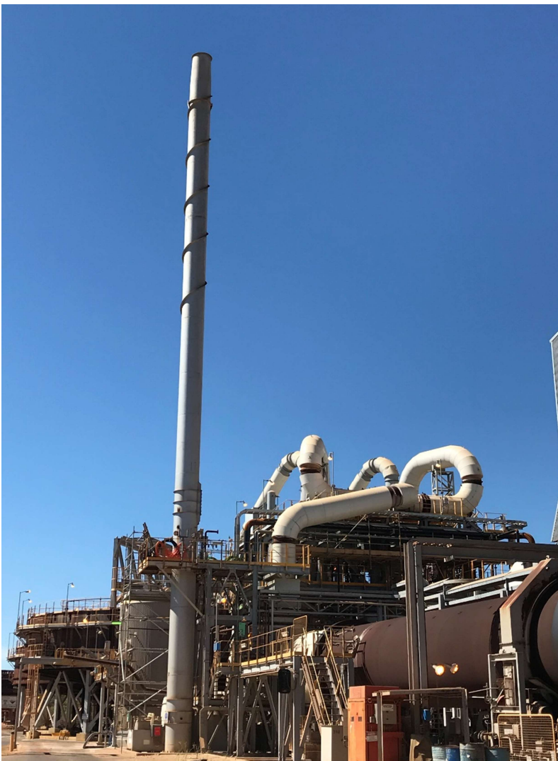
Figure 10: Oxalate Kiln RTO Stack
