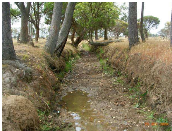
Plate 8. Ferraro Brook reach, benchmark #1, cross-section #3; downcut banks, exposed tree ( Eucalyptus rudis ) roots.
