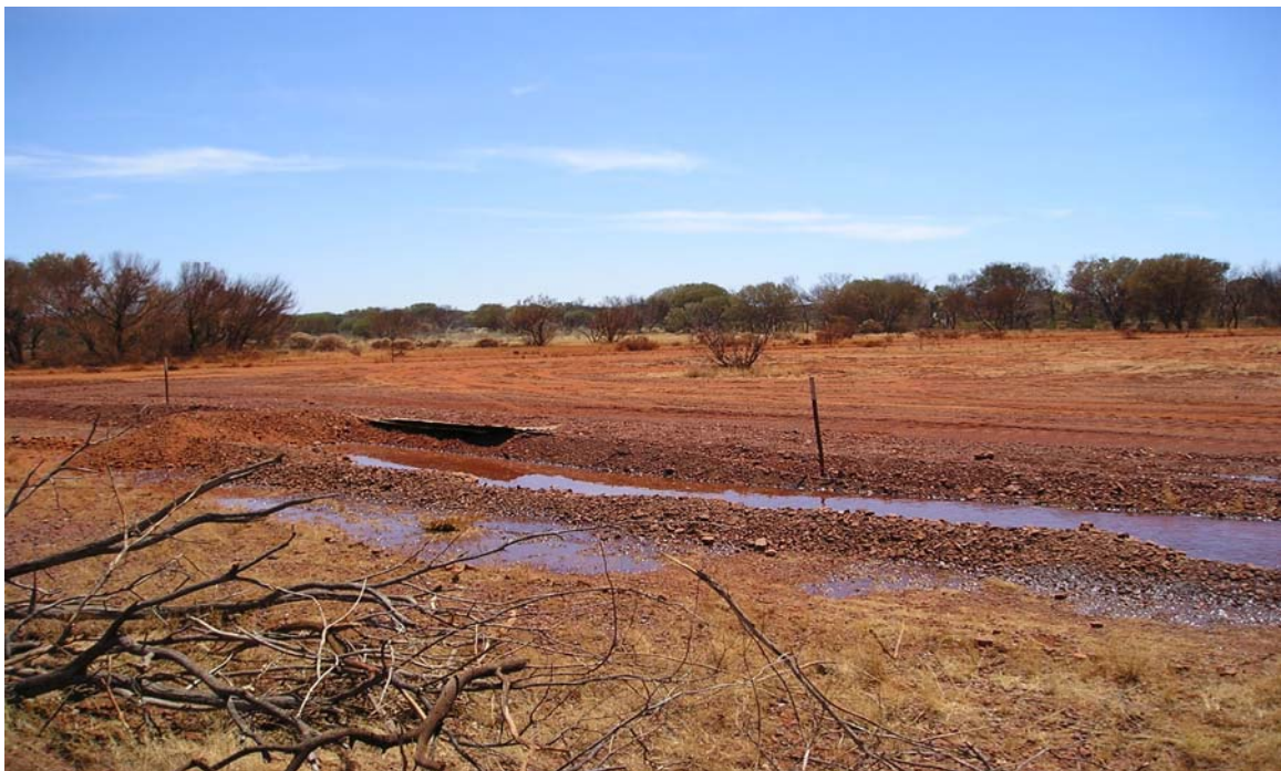
Fig 15: "Top" levee. The front levee was constructed quickly with a loader. The original levee in the rear was too wide and consolidated for the purpose. Permeability was not uniform, but the levee leaked in sufficient places that continuous sheet flow was quickly established.
