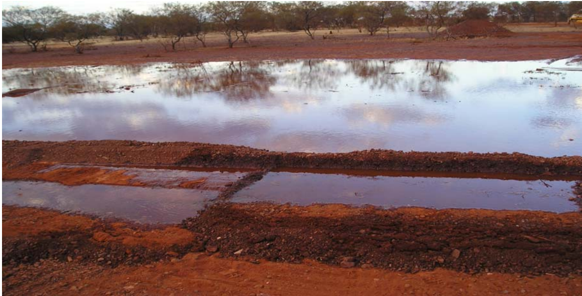
Fig 14: "E20 Levee". This had a high proportion of very fine material, and insufficient permeability, and it is likely it would have eventually over-topped with sufficient water. Effective at spreading the water.
