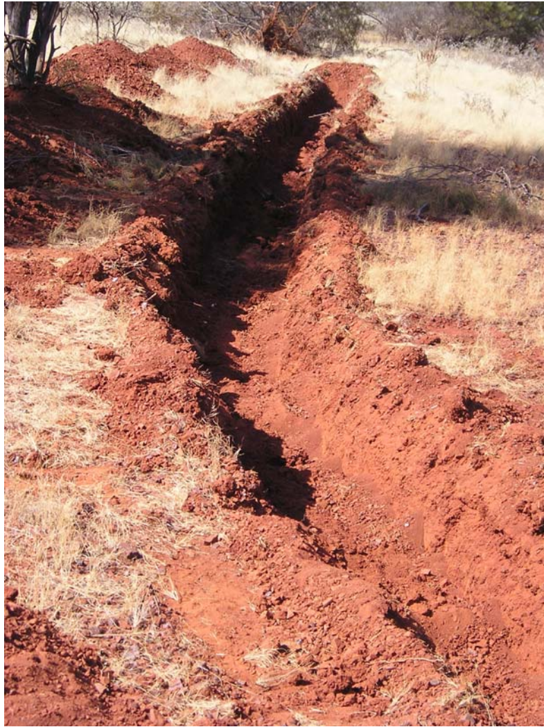
Fig 10: Minimal disturbance of natural surface to retain level. Spill removed by hand.
