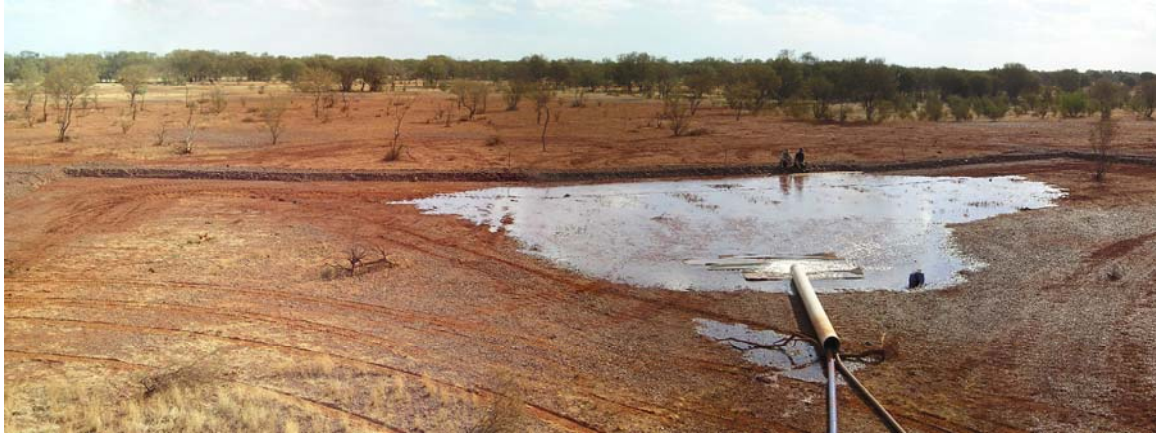
Fig 5a: E20 Levee site facing south. The “head” has reached the levee wall. Further spread is initially along lower areas back from the wall.
