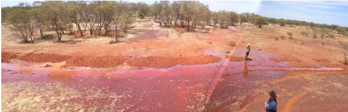
Fig 8: Spreader ditch with bund on down slope side. Note the breaks in the bund in the centre and left of the picture have been affected by cattle trampling, with the one in the centre of the picture completely closed.
