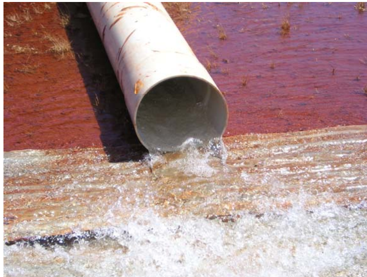
Fig 1: Use of corrugated iron to dissipate energy. Flow rate 23 litres/second.
