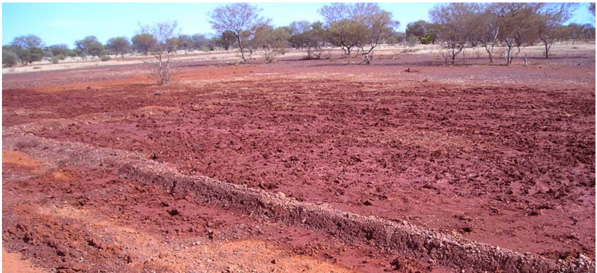
Fig 13: Cattle trampling did not materially affect the levee bank.
