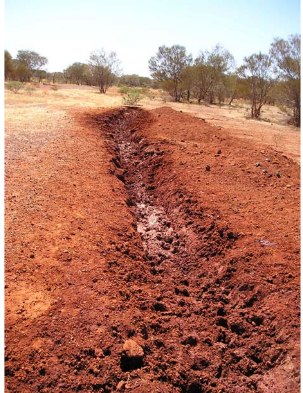
Fig 12: Cattle damage 24 hours after filling.
