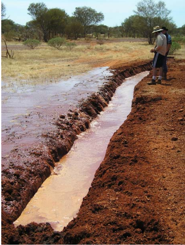
Fig 11: Ditch edge may need armouring to prevent erosion.
