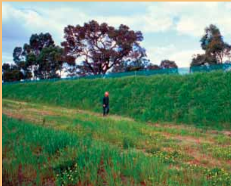
An example of a topsoil bund wall
