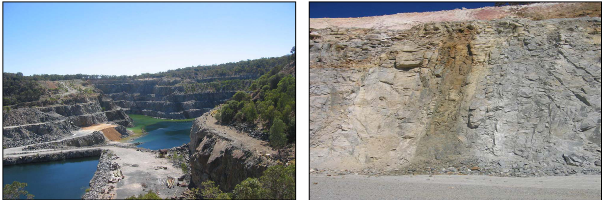
Plate 9 Impermeable dyke at former Herne Hill Quarry (left) and seepage from granite fracture at Red Hill Quarry (right)
