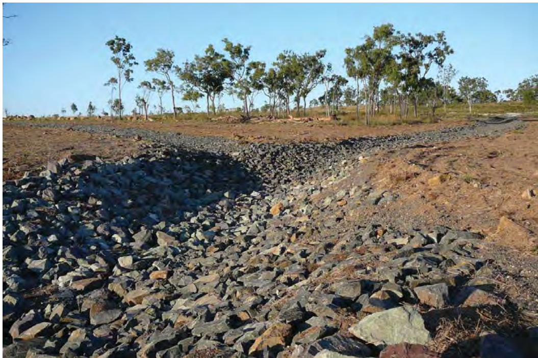
Armoured rock chutes for drainage erosion management: a potential feature of Yandicoogina landform designs
