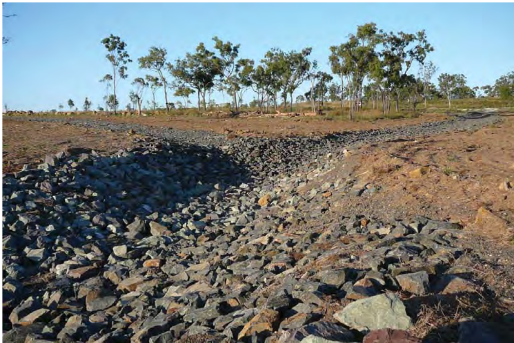
Figure 33 Example of a rock chute structure used to control water ingress into the channel
