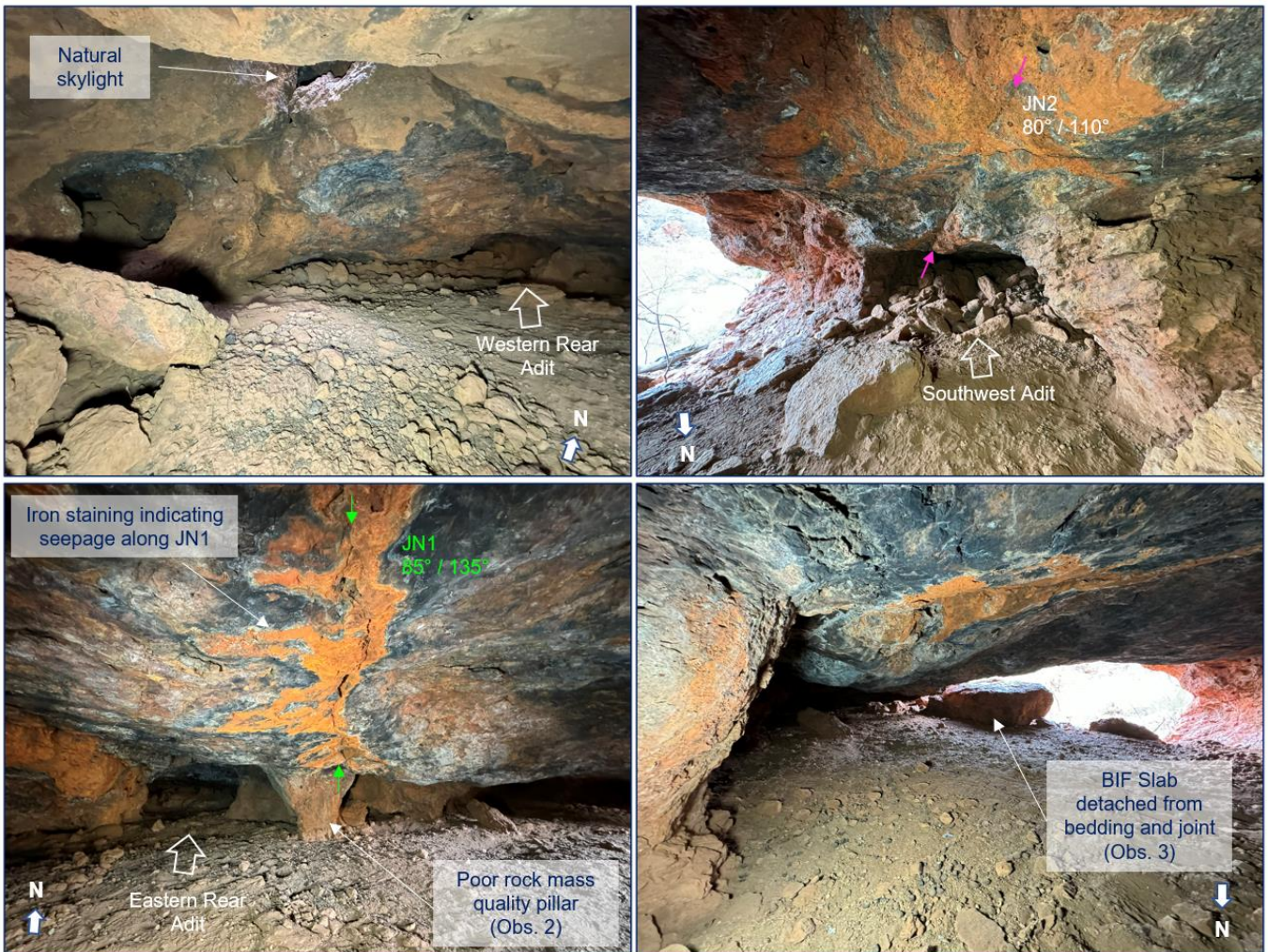
Inset 13: Engineering geological observations of cave MEC016 (MIB-MD13-043) interior. Top Left: Cave interior viewed towards the northwest showing access point to the western rear adit and the natural skylight developed in the cave roof. Top Right: Interior viewed towards the south showing cave entrance and access point to southwest adit. Bottom Left: Joint set 1 intersecting the interior roof, and access point to eastern rear adit. Bottom Right: Cave interior viewed towards the south showing a large slab detached from bedding in the cave roof.
