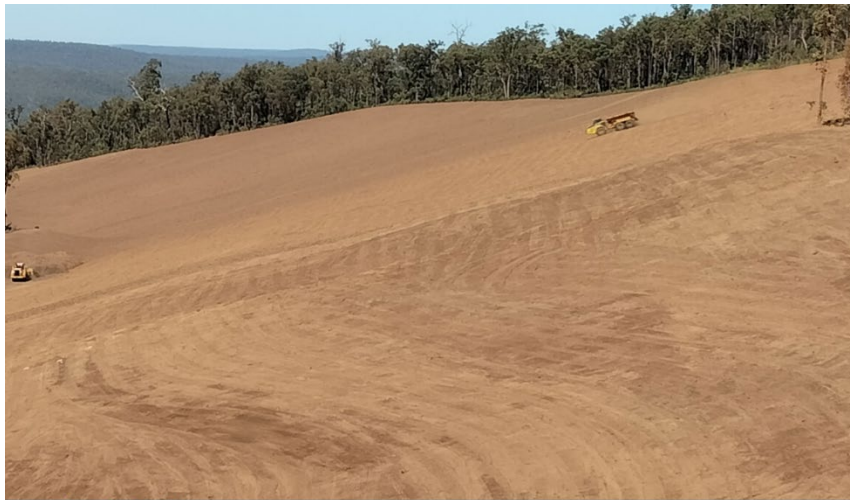
Figure AA-12: Landscaping completion and Fresh Topsoil Return
