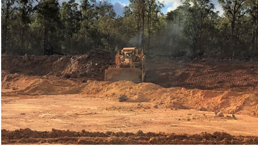
Figure AA-8: Landscaping - vertical pit face reshaping and blending
