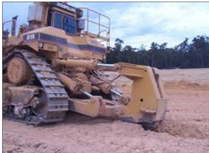
Figure AA-7: Pre-landscape ripping
