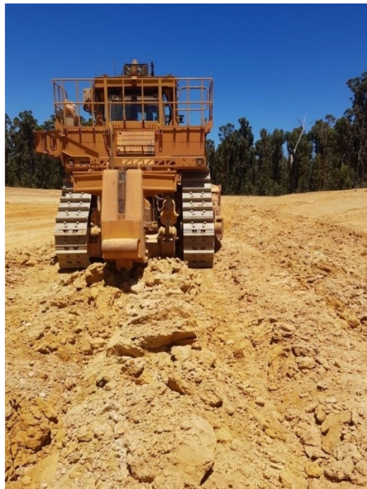
Figure AA-9: Post-landscape ripping
