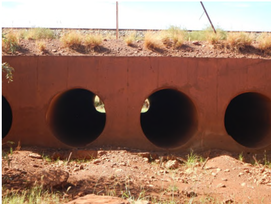
Figure A.48. Upstream view of 1500 mm culverts underneath the Rio Tinto railway and access road crossing of a tributary to Caves Creek. Note the presence of calcrete in the foreground.
