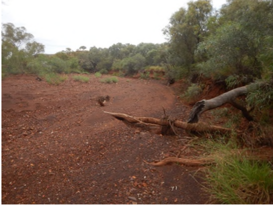
Figure A.13. Bank erosion along the right bank of Pinarra Creek in SR P4.
