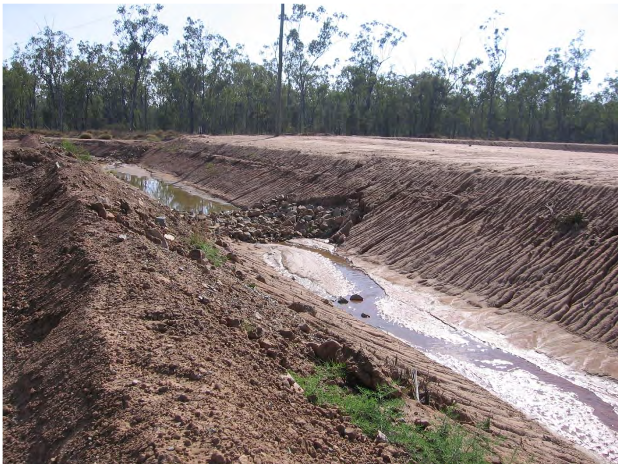
Figure 22: Example of drain batter erosion in a sodic soil in Queensland.
