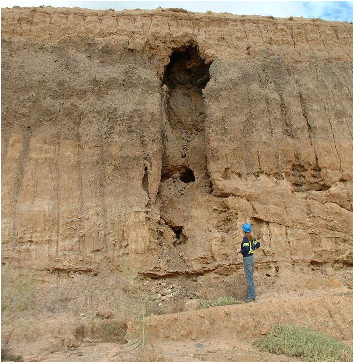
Figure 20: Sodic soil batter in Queensland.
