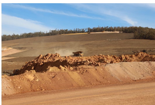
Photo 9 Myara Mine Region, with haul road and rehabilitation activities underway
