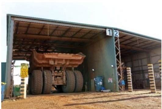
Image: Supplied by Alcoa Photo 20 Vehicle fuel bay
