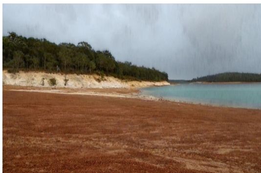
Photo 5 Southern edge of Logue Brook Dam
