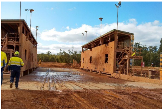
Image: Supplied by Alcoa Photo 22 Vehicle wash bay
