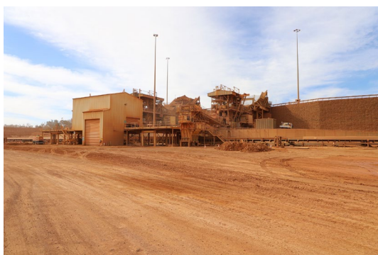
Photo 7 Example of crusher (Myara Mine Region)
