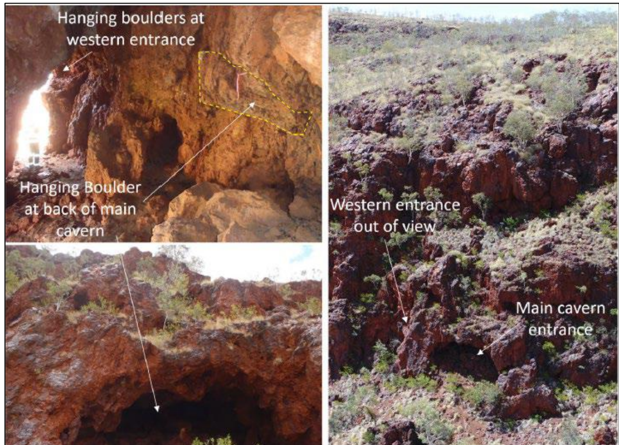
Figure 9 CMRC-15 potential failure locations (PSM 2019)
