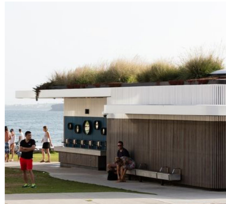
Hub Green Roof
