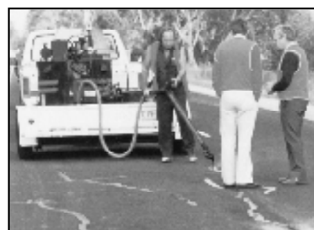
Filling and sanding cracks after routing
