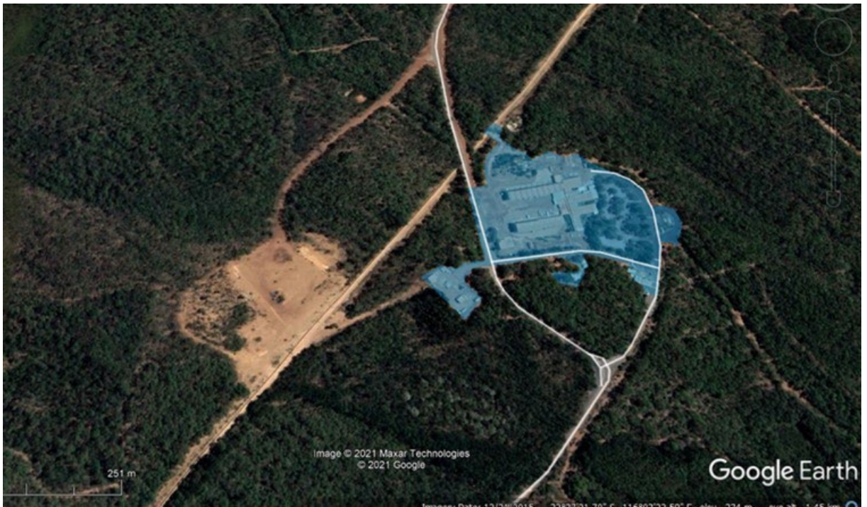
Plate 2-4 Main Huntly facilities
