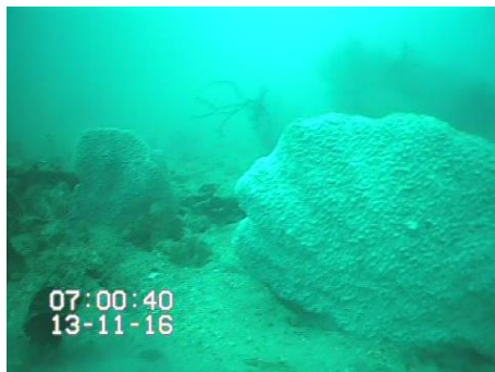
Plate 3 Observations of the marine environment at the base of the ship loader piles and growth on the piles
