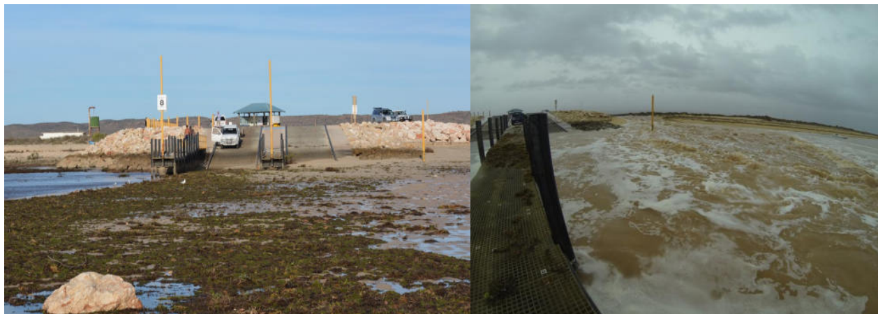
Figure 4 Flooding of Tantabiddi Creek and sedimentation at the boat ramp caused by the April 2014 flood
