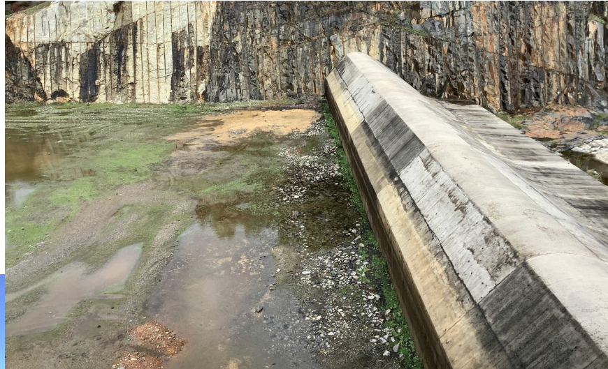
Photo 7. Example of a concrete crest block to deter W1-SP0 access
