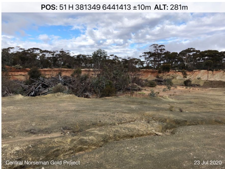
Existing borrow pit near proposed ROM
