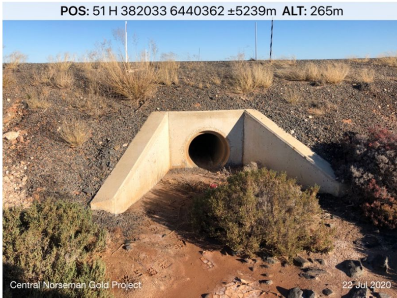
Culvert below Coolgardie-Esperance Highway
