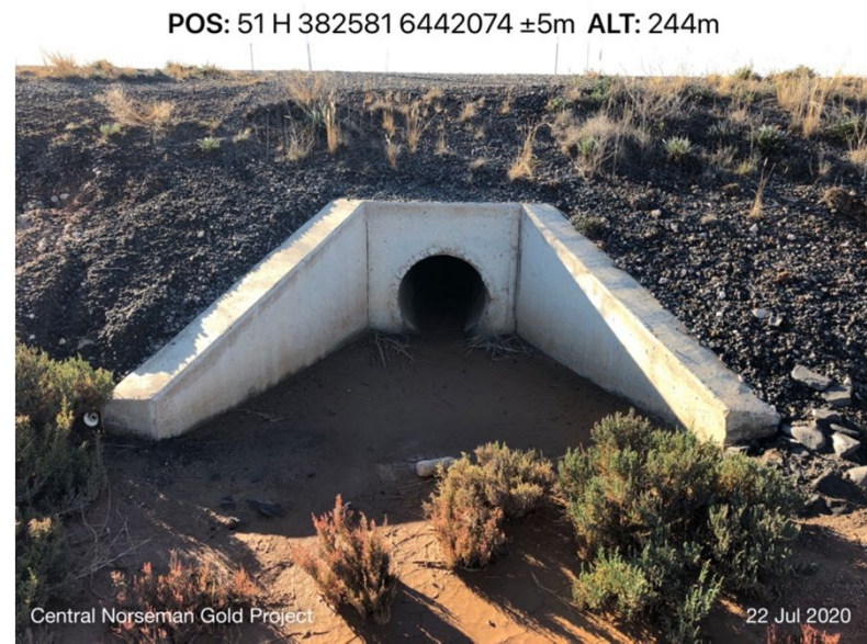
Culvert below Coolgardie-Esperance Highway
