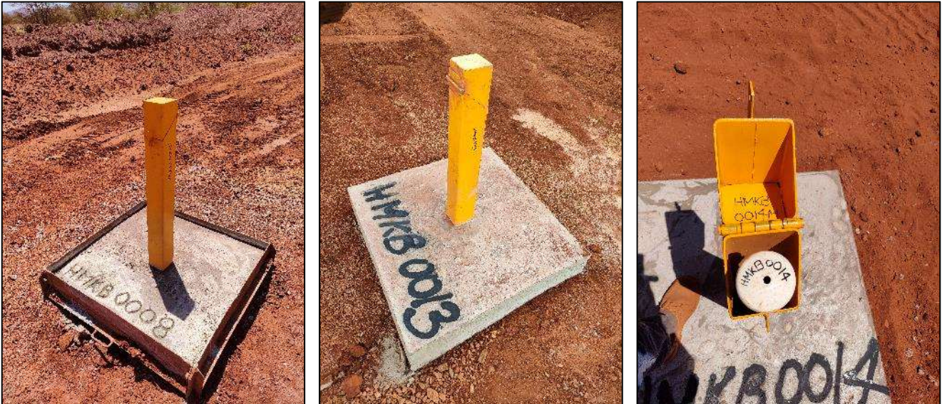
Figure 5, 6 and 7: Monitoring bore completion with vented lid
