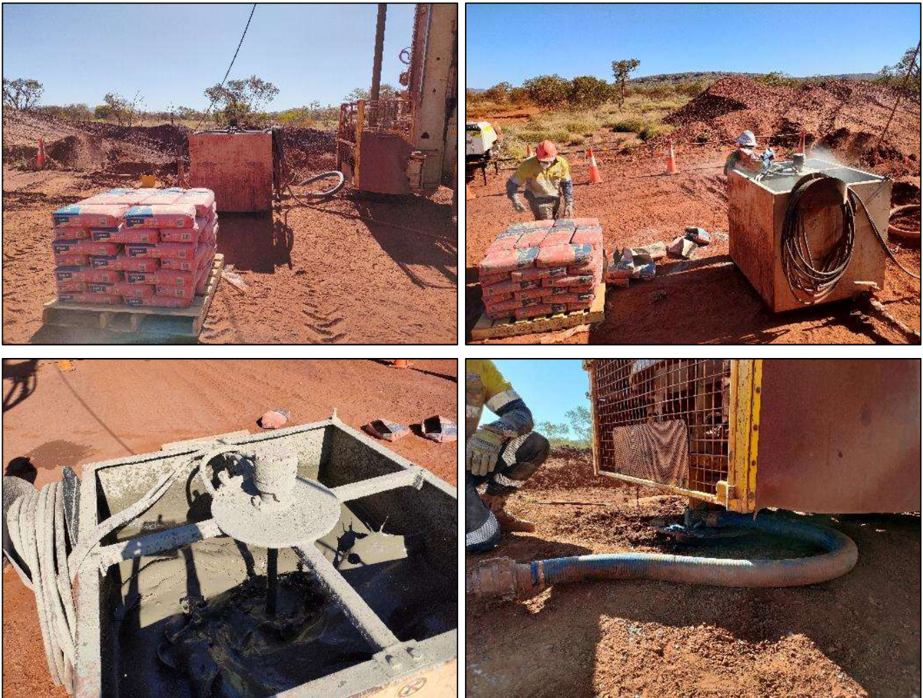
Figure 23, 24, 25 and 26: Grouting and Mixing Operation
