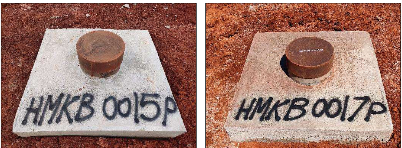
Figure 8 and 9: Production bore completion
