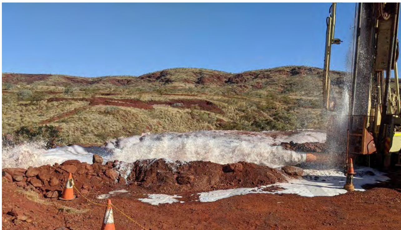
Plate 5: Final reaming of HMN0003 with extensive use of drilling foam
