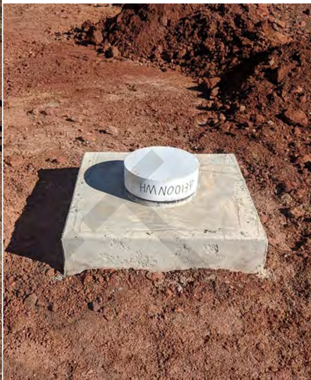
Plate 2: Typical headworks completion of the production bores (HMN0013P)
