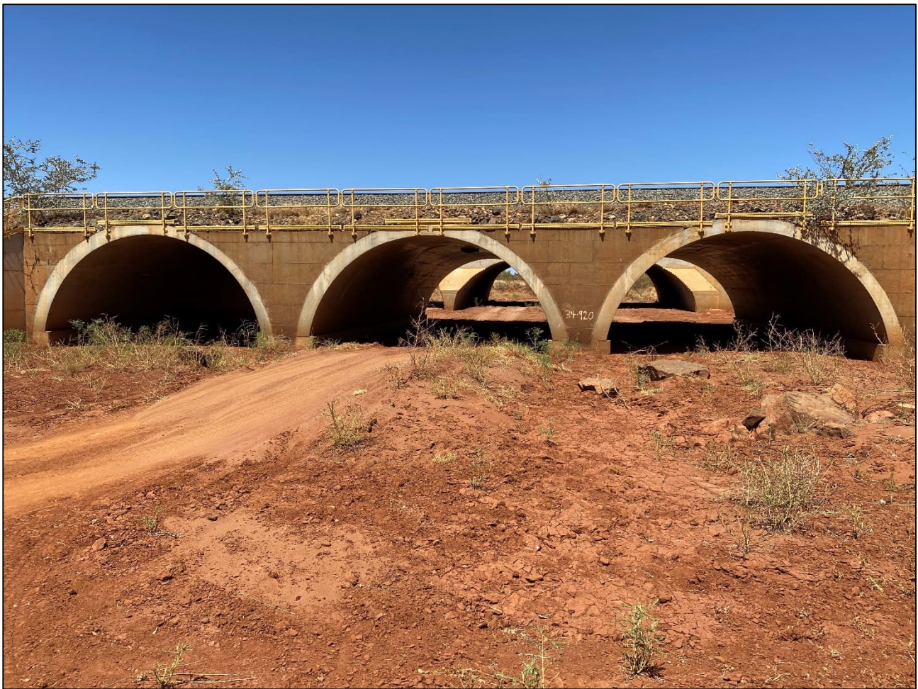
Figure 5-1: Example of arch structure with alluvial bed located on Rio Tinto Iron Ore Railway
