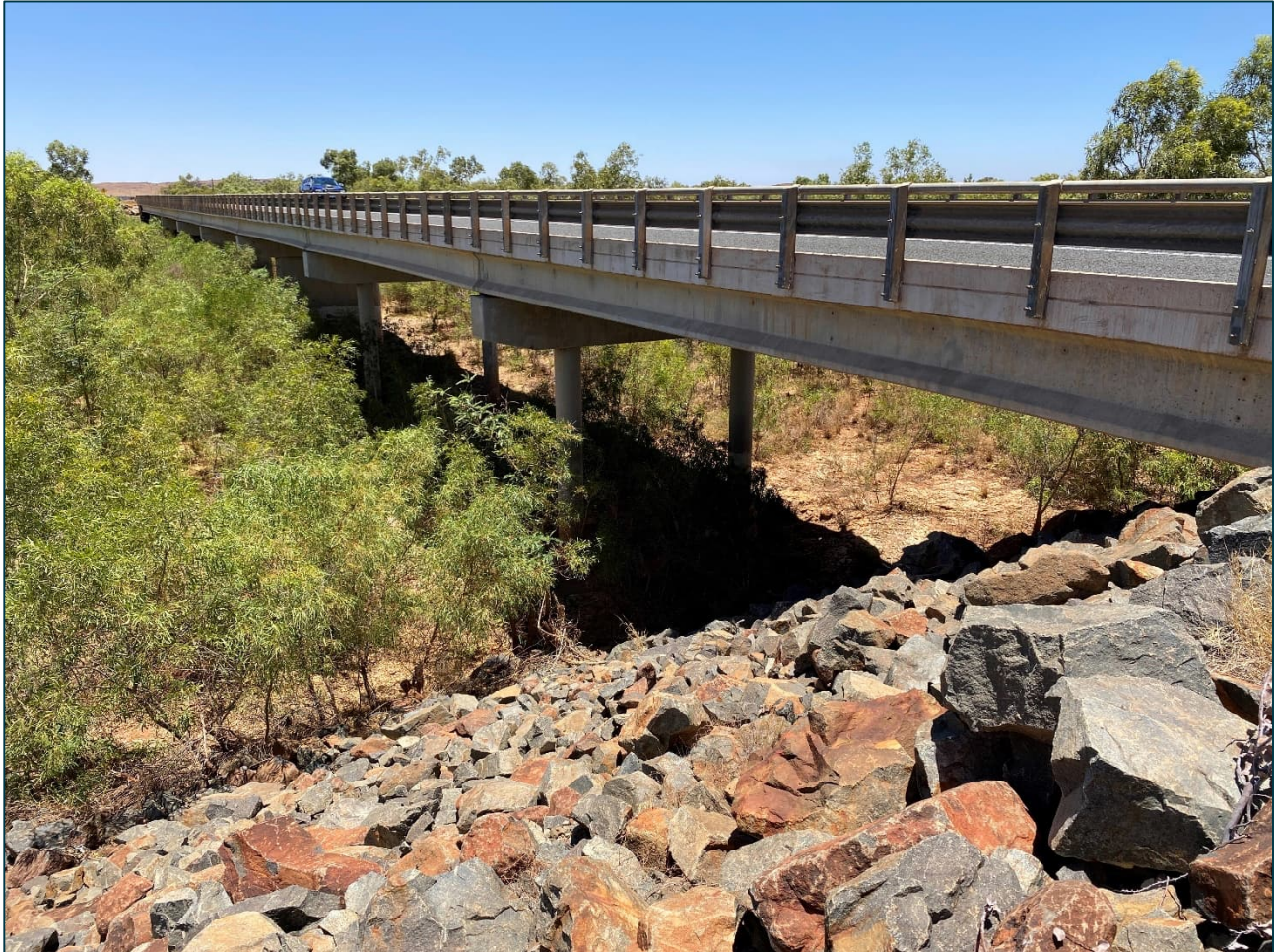
Figure 5-2: NWCH bridge crossing of Harding River at Roebourne
