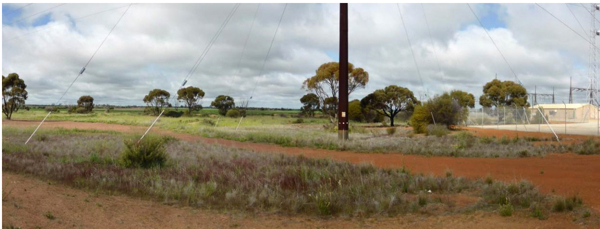
Figure 5-1 Proposed substation site, showing highly disturbed, degraded vegetation of Type A(vd). Photo taken from Habitat Plot 29.
