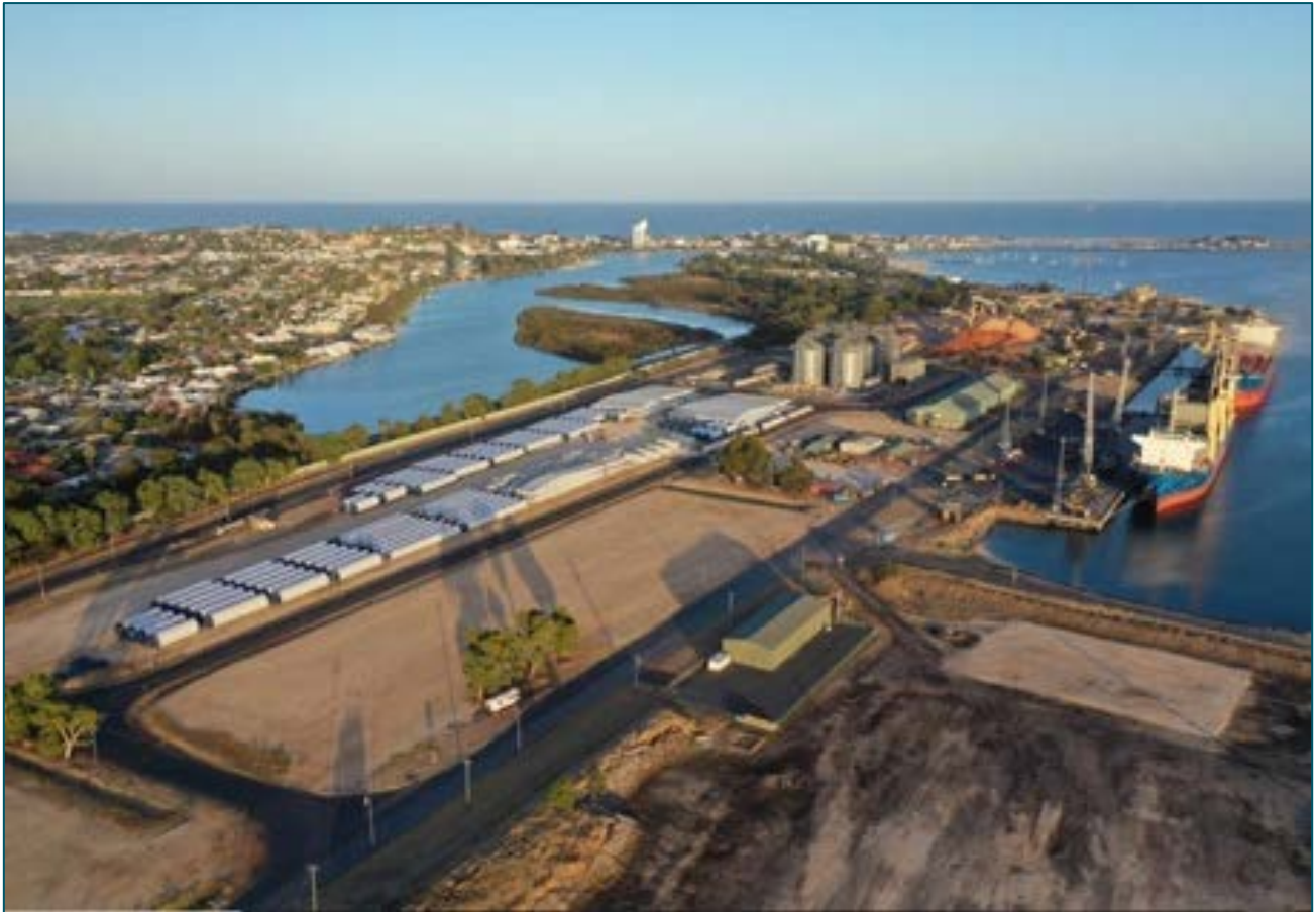
Figure 6: FRWF1 Turbine Components Unloading at Port of Bunbury
