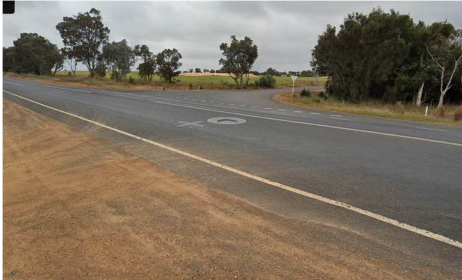
Figure 19: Albany Highway onto Shamrock Road
